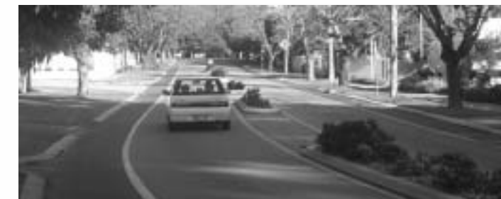
Contrast coloured bikelane between kerb and vehicle lane provides safe space for cyclists.
