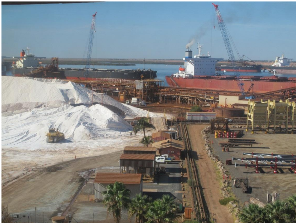
Port Hedland Port—on the left salt stacked for shipping is moved with a bulldozer; on the right ships enter the port for loading.
