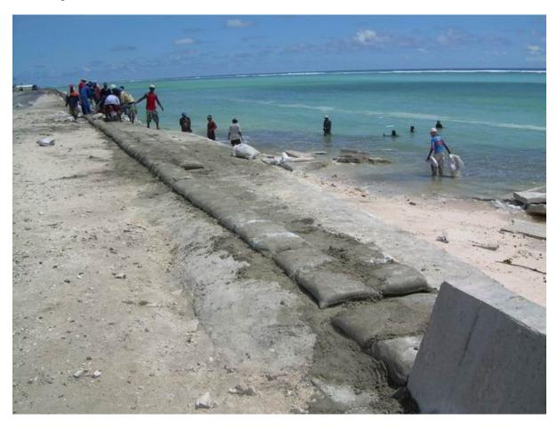
Rising sea levels and flooding cause damage in low-lying islands of the Pacific. Here people in Kiribati are repairing a breakwater damaged by strong currents (image courtesy of the Pacific Calling Partnership at the Edmund Rice Centre).
