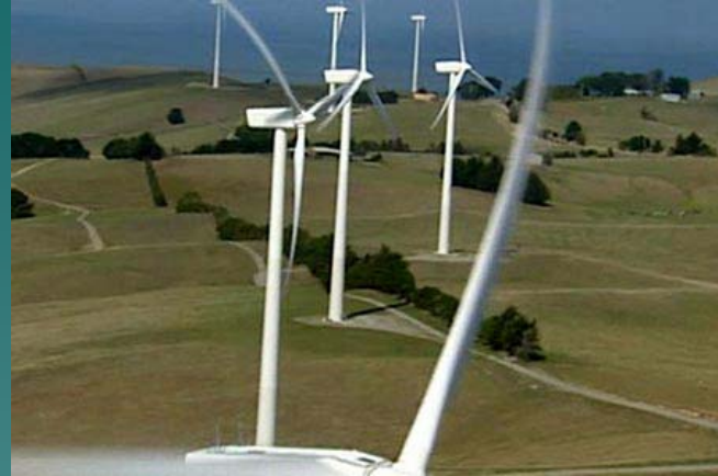
329 Megawatt Macarthur wind farm, VIC.
