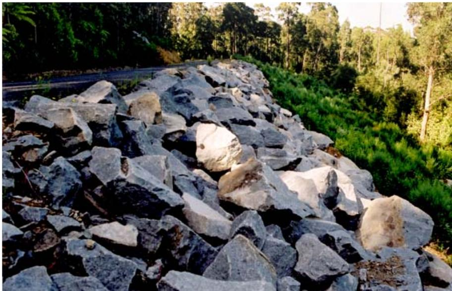
Figure 8.4.6 Quarried Rock stabilizing the South Face Road where erosion has occurred
