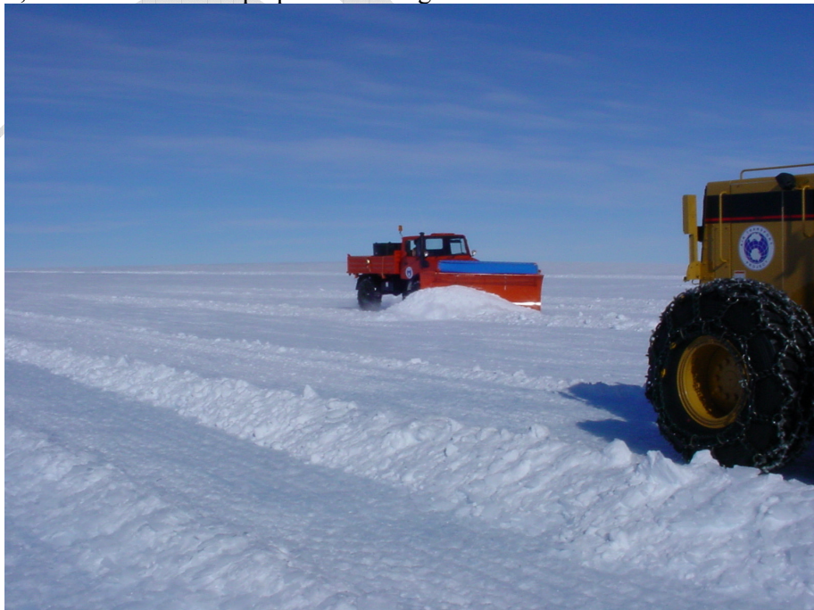
Photo 3: Trial runway construction 2002/03 (George Blaisdell)
