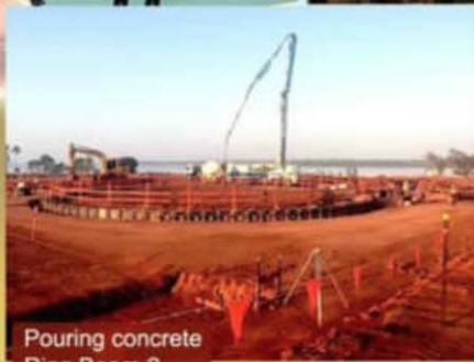
Building the Tank Farm walls
