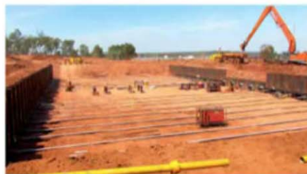
Biggest crane ever on Tiwi Islands
