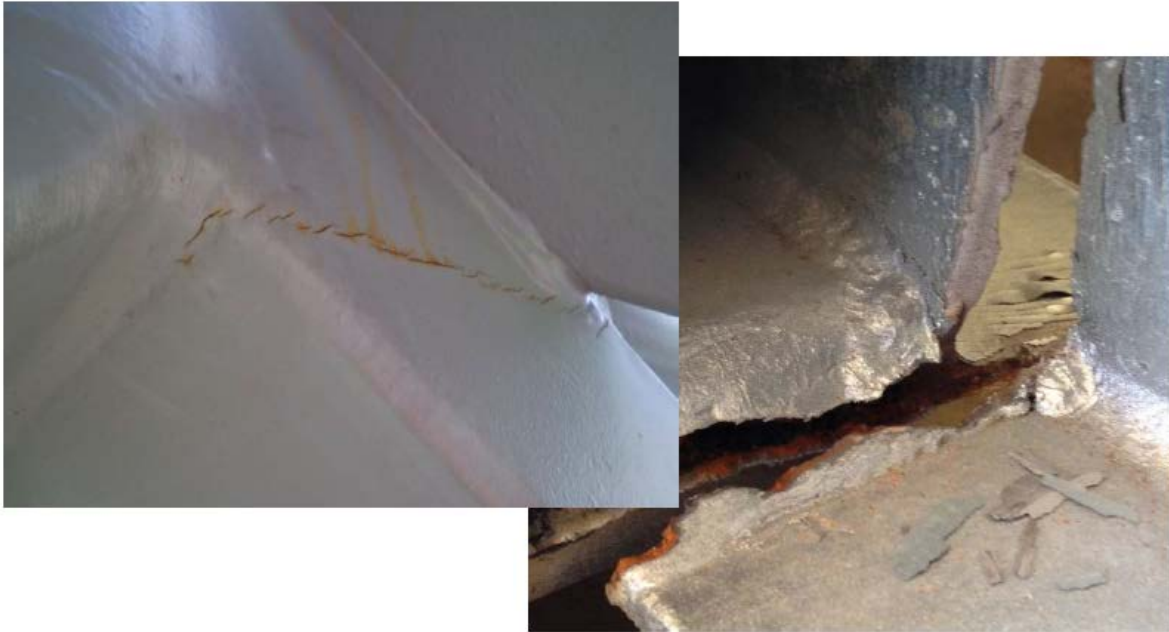
Figure 4.2: Steel cracking on imported fabricated product 49
