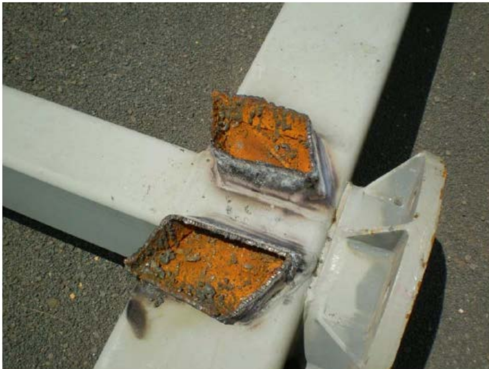
Figure 4.3: Diagonal chords on a bridge truss filled with water 50
