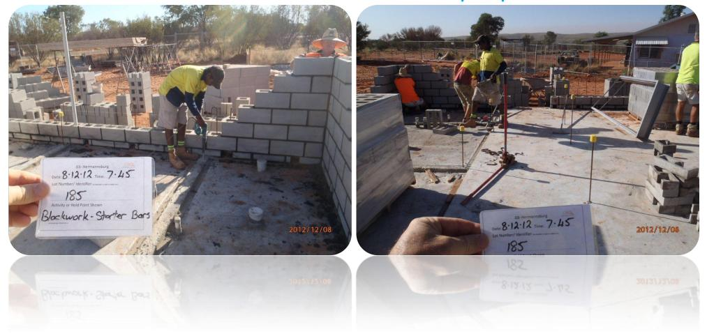
NFA apprentice Wayne Patrick drilling and placing starter bar ready for the block workers.
