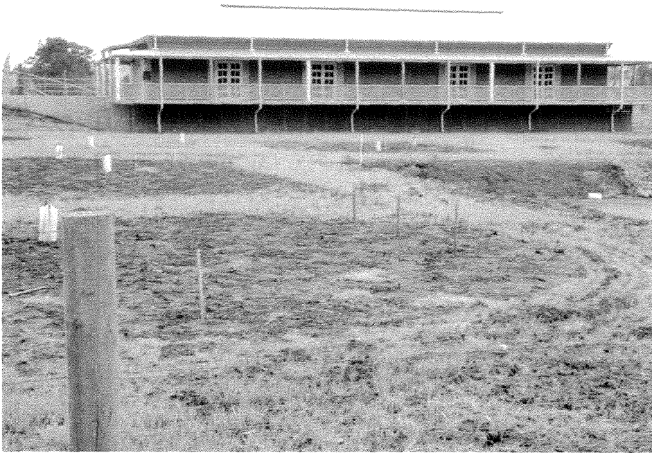
No, not a house but the pump shed on the Heritage listed Goulburn River for the North South pipeline in disguise! Nov 2010
