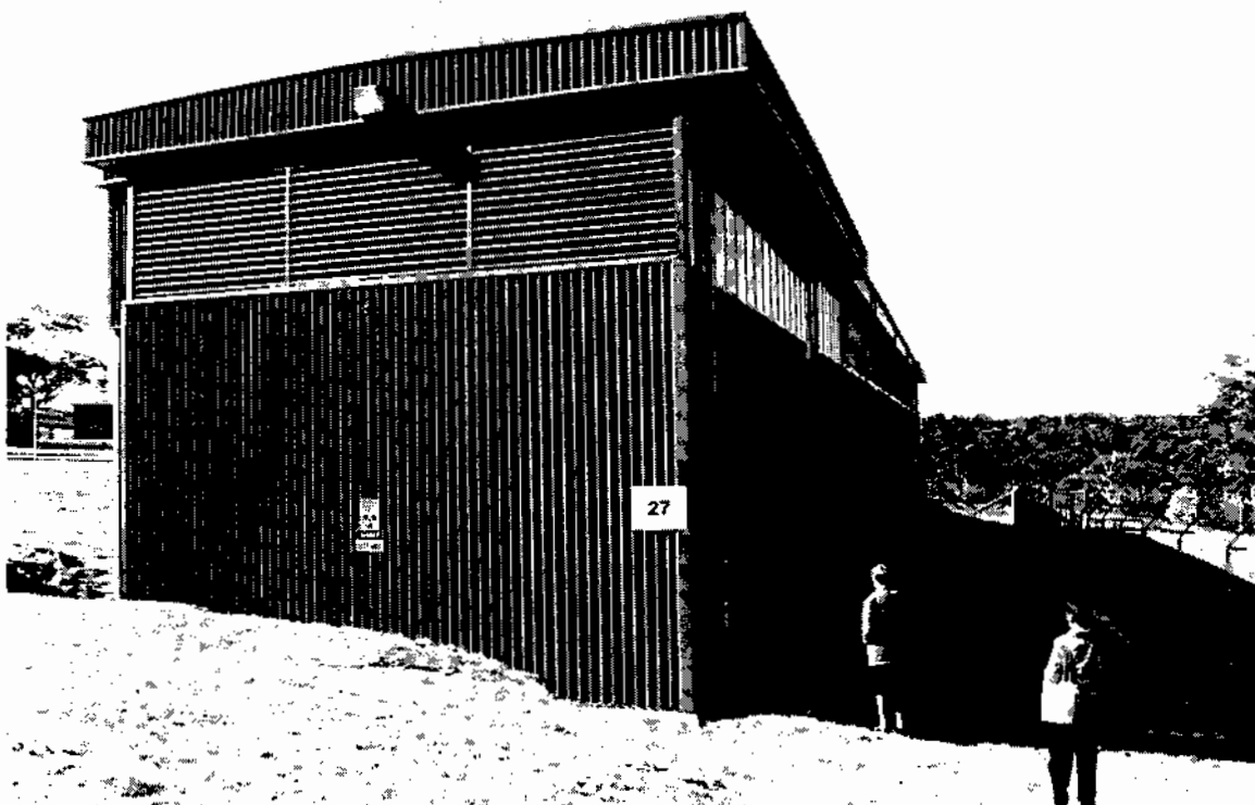
The building containing the spent fuel dry storage facility and the solid intermediate level waste storage facilities (Photograph provided by ANSTO)
