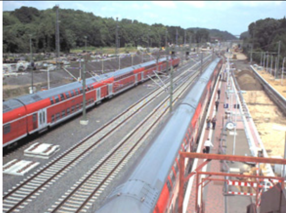
↑ Example of quadruplication work between Cologne & Brussels
