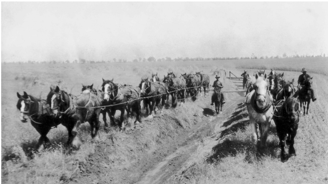
Fred Stillard, constructing earth for the original irrigation channel in the area.
