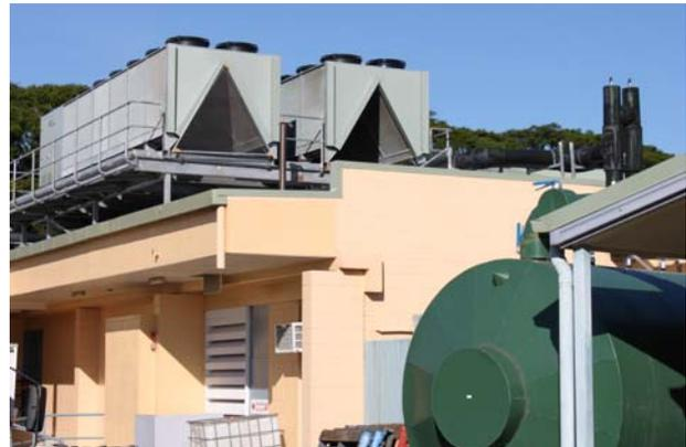
Thermal Energy Storage tank (at bottom right) with air-handling units above.
