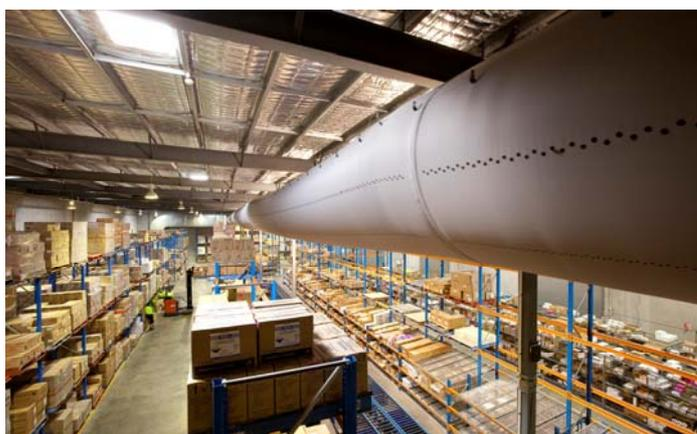
Above: Cooled air is circulated via a fabric duct hung from below the ceiling.
