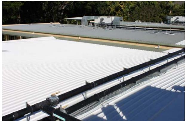
**The temperature on the near roof painted with heat-reflective paint is 18° cooler than the far roof yet to be painted.**
