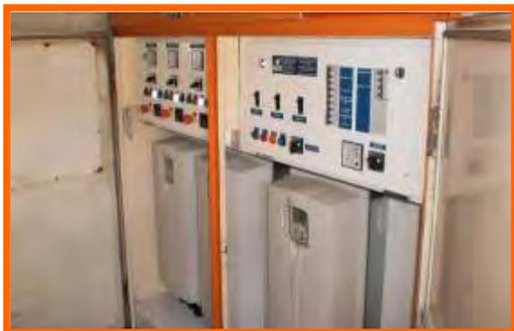
*New switchboard with variable speed pump drives*
