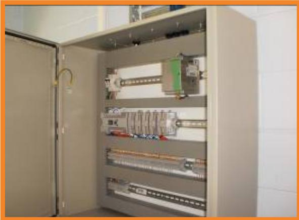
*Installing an air conditioning control system featuring Allen Bradley hardware resulted in a 25 per cent running cost reduction. It can shut down the air conditioning when a window or door is opened for any length of time.*
