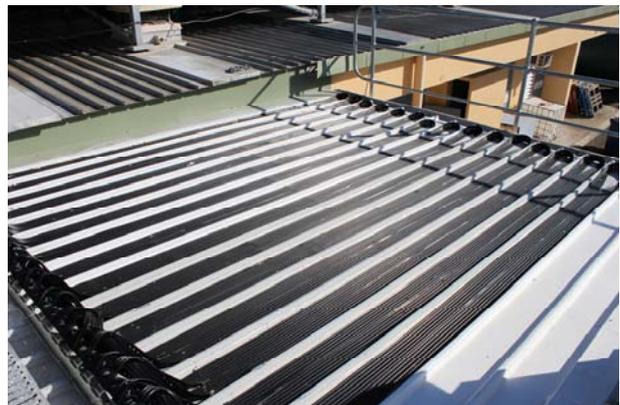
**The DIY solar water heater uses pool blankets coiled on the rooftop.**
