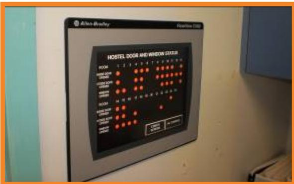
*The new user interface, hardwired back to the control box above, allows staff to easily determine status of each unit's air conditioning and control how the air conditioner will operate.*
