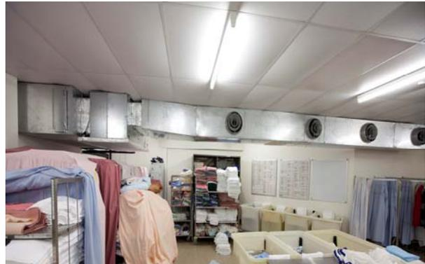
**Chilled water is used to air-condition the home's large laundry, saving a significant amount of energy over conventional DX air-conditioning.**
