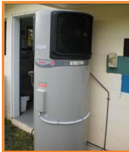
*Heat pumps reduced the energy used to heat water by 70 per cent.*
