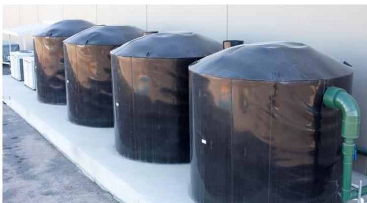
**The thermal energy storage tanks effectively operate as a battery in the system, allowing the building cooling system to be decoupled from the process plant.**
