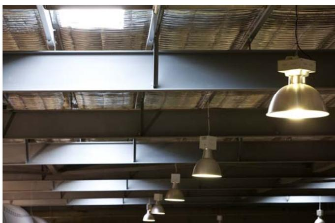
Above: The hi-bay lighting automatically switches off when there is adequate natural light penetration through the warehouse skylights.
