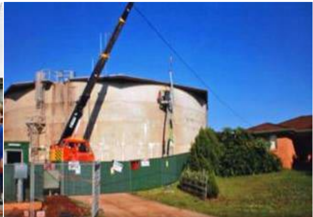
Image 2: Optus starting construction
