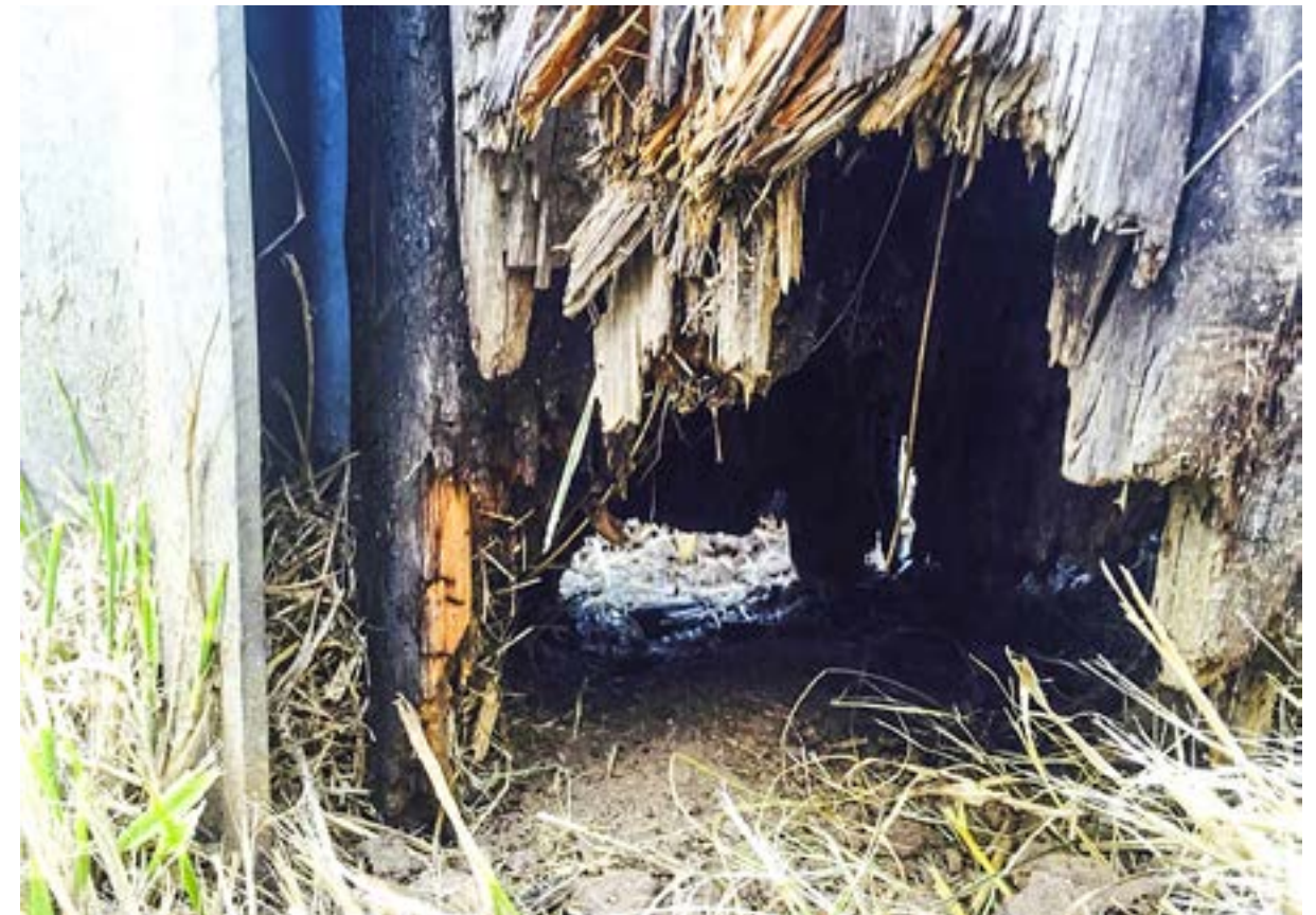
✖ Pole in service - completely rotten on ground.
