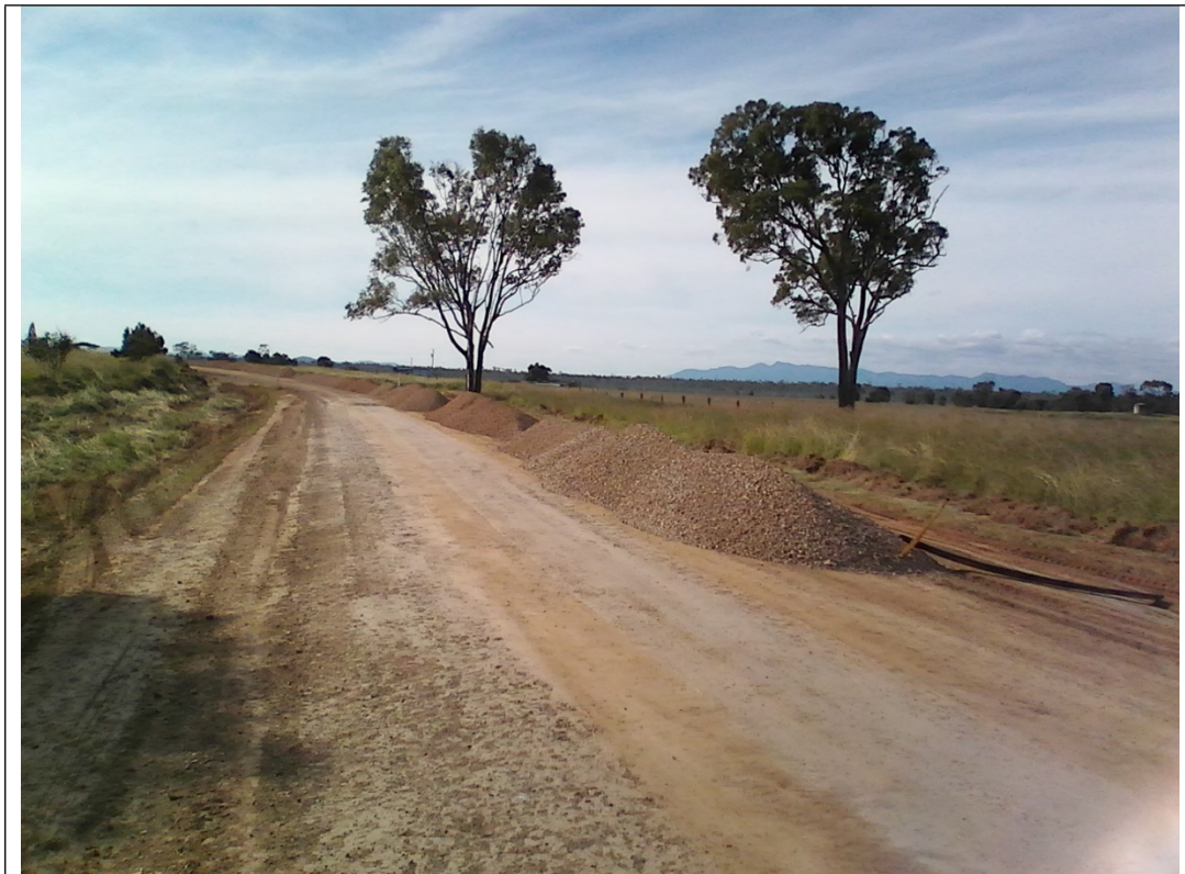
Figure 1. Gravel top dressing on road in the Fitzroy catchment of central Queensland. This was a continuous line of dumped material for 2km of a 4km stretch of road.
