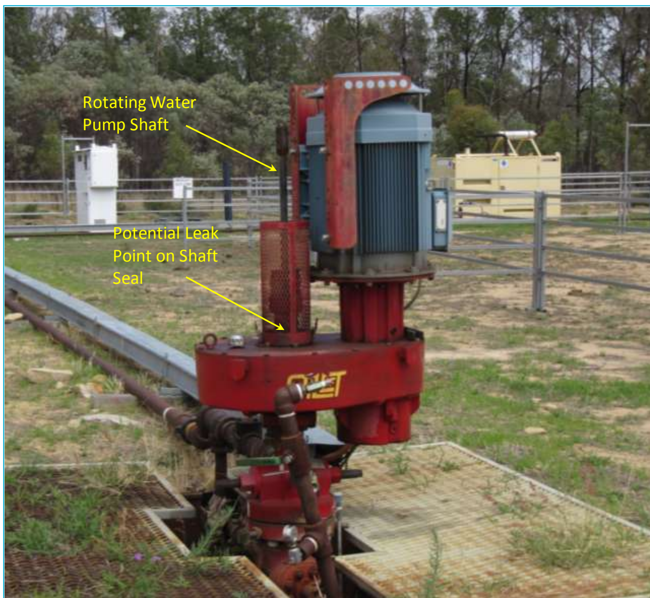
Figure 5.3. Well head showing the location of the water pump shaft and seal which was found to be a common leak point.
