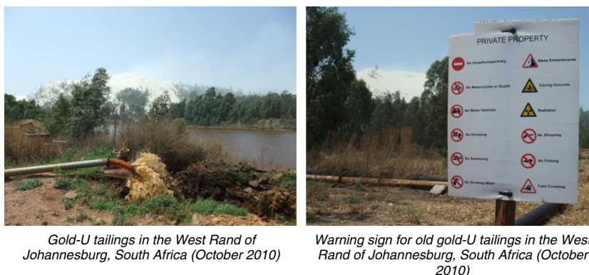
Fig. 12. A tailings dump in the West Rand, Witwatersrand Basin, South Africa, showing wind-blown erosion from the top and acid mine drainage in the foreground (photo's author).
