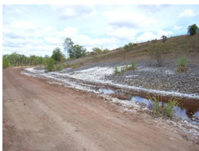
Acid mine drainage (AMD), containing acid, salts, heavy metals and radionuclides, leaking from White's waste rock dump, Rum Jungle, Australia (July 2007, ~21 years after rehabilitation)
