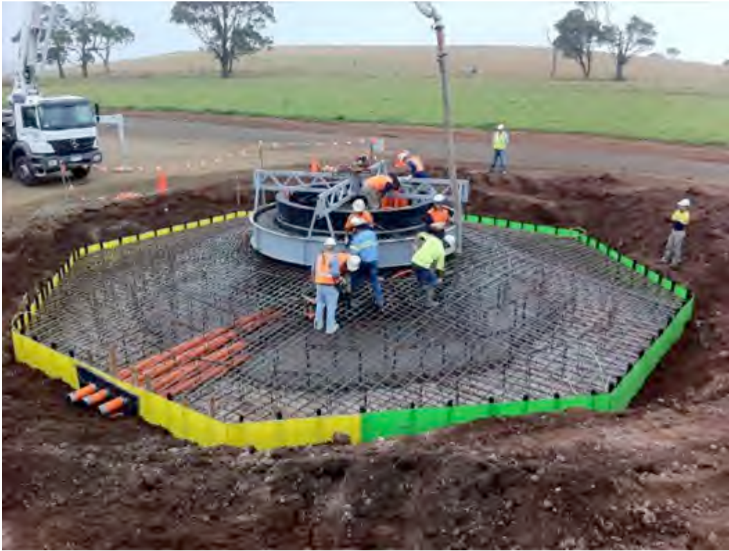
Construction of the first wind turbine foundation at Leonards Hill, February 2011
