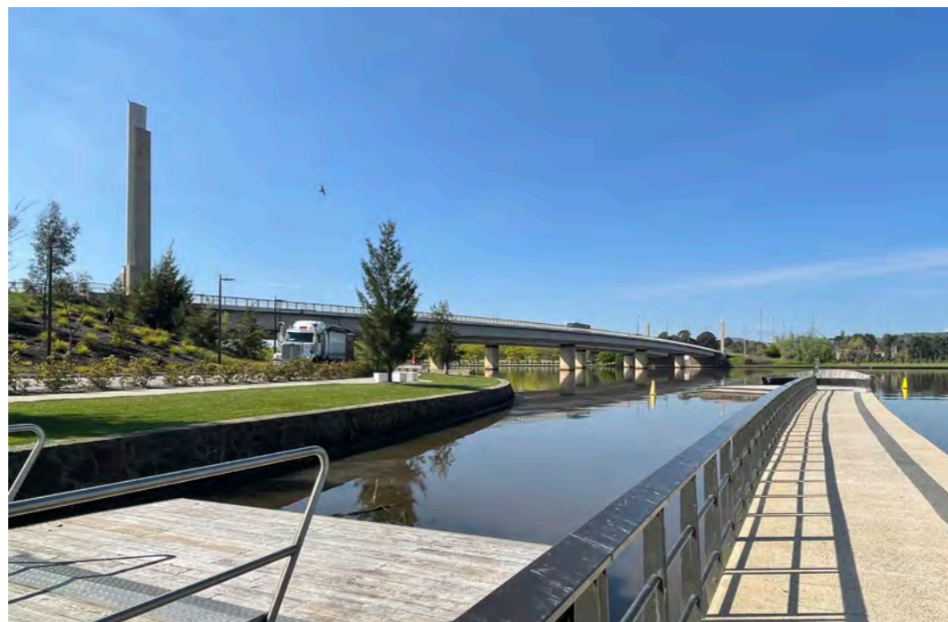
Figure 120: Commonwealth Avenue Bridge viewed from Henry Roland Park
