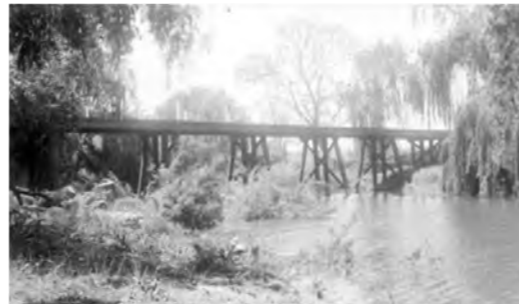
Figure 10: 1921-22. Old Commonwealth Avenue Bridge over Molonglo River destroyed in July 1922 floods. Source: National Archives of Australia, A3560, 232, Item ID 3106888.
