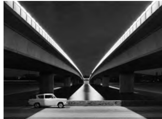
Figure 69: 1964. Commonwealth Avenue Bridge crossing Lake Burley Griffin.
