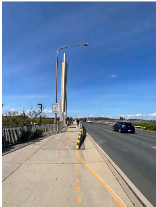
Figure 144: Approach to bridge southbound.
