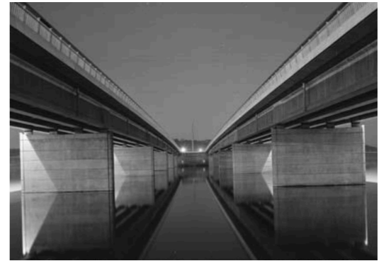
Figure 72: 1964. Kings Avenue Bridge 22.5.1964.
