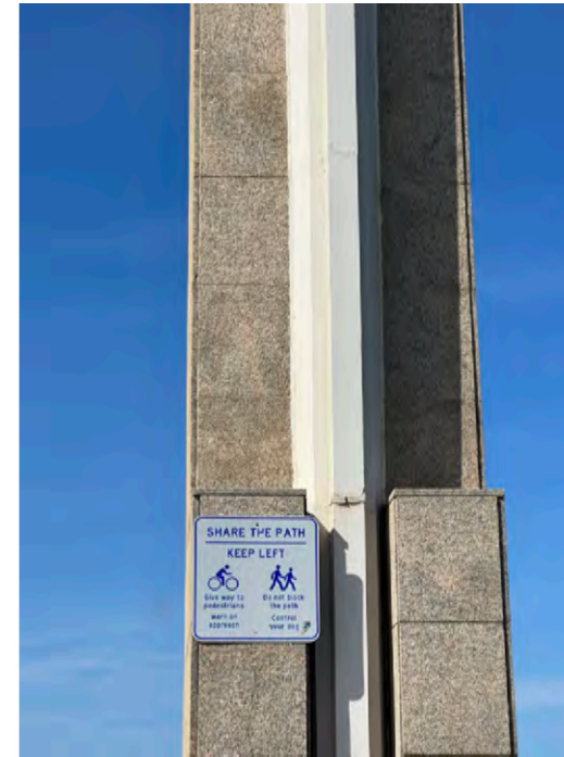
Figure 196: NW Pylon detail.
