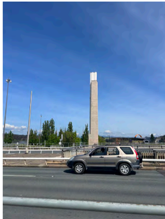
Figure 157: SW Pylon across lanes.
