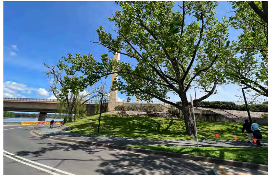
Figure 137: NE Pylon and stair from across Barrine Drive.
