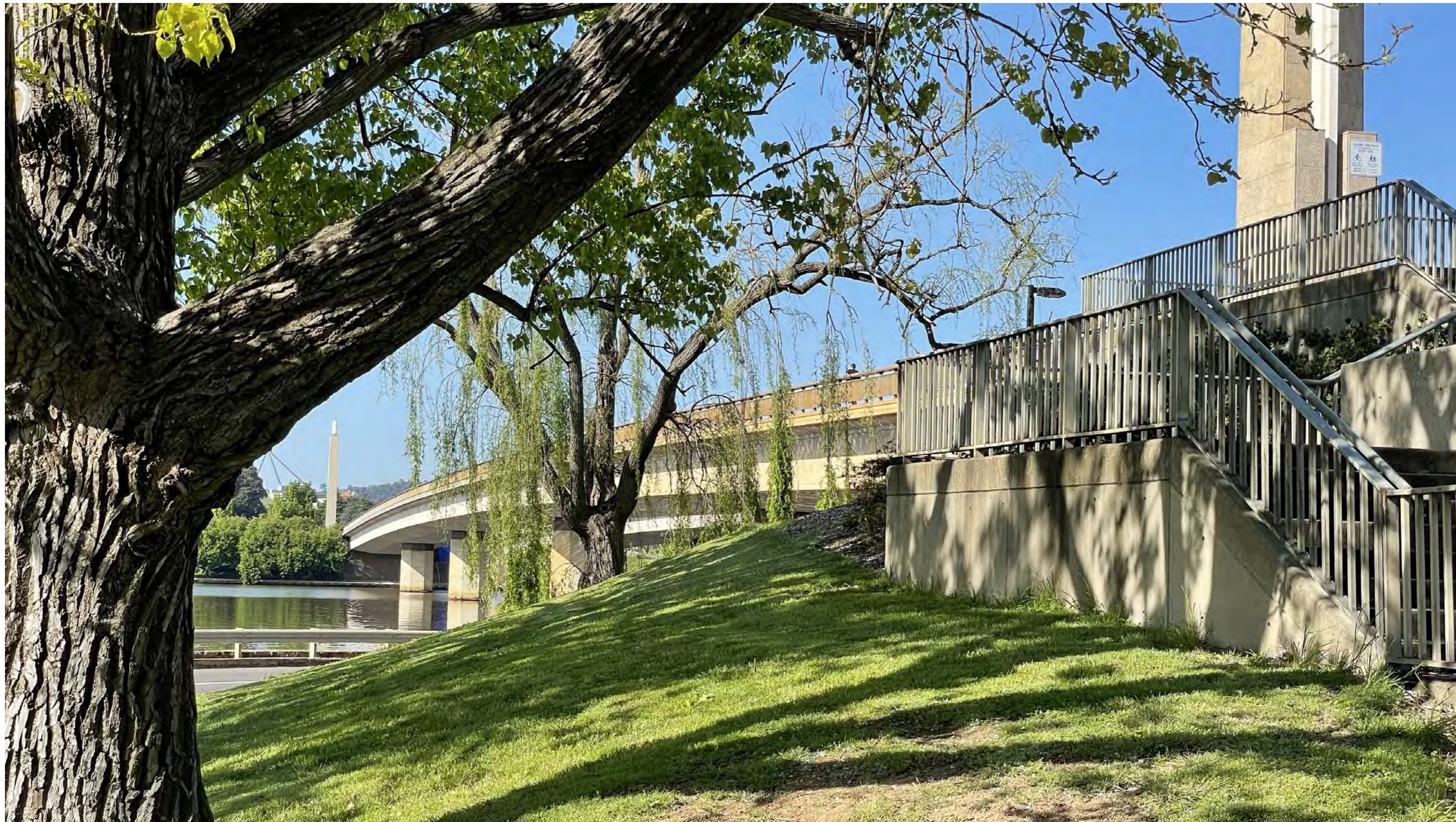
Figure 40: Views of Commonwealth Avenue Bridge from the northern side looking south
