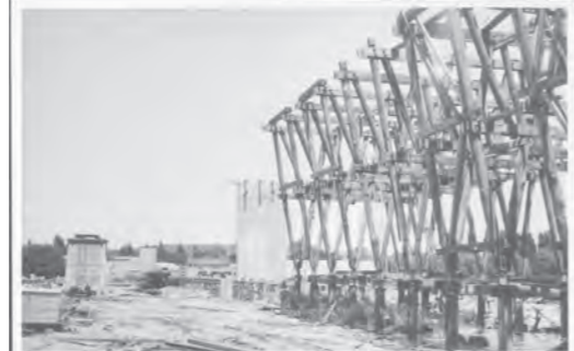
Figure 56: 1962. Commonwealth Avenue Bridge under construction, 1962 or 1963, 6 [picture]. Source: Trove, https://nla.gov.au:443/tarkine/nla.obj-145674973
