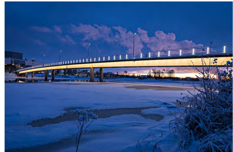
Precedent Image – Pikisaari Bridge – City of Oulu – Finland Bridge Panels illuminated with warm white luminaires
