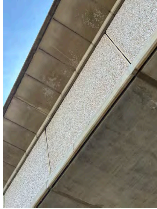
Figure 131: Detail shot of bridge edge showing precast panelling.
