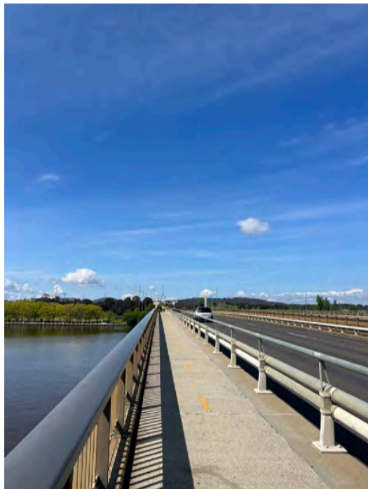
Figure 153: Pedestrian/ Cyclepath southbound.
