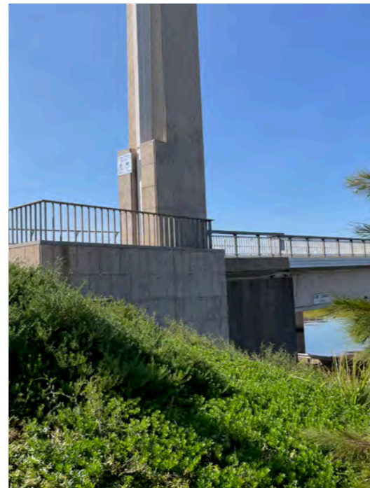
Figure 123: Base of Pylon situated NW of bridge.
