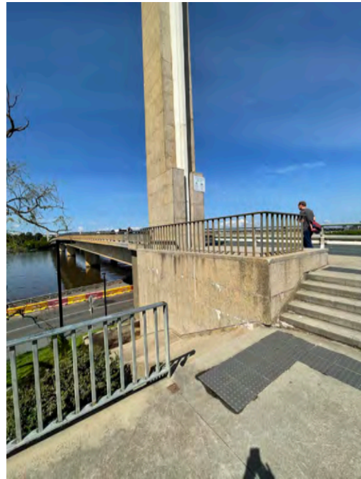
Figure 140: Stair arrangement around plinth to pylon.
