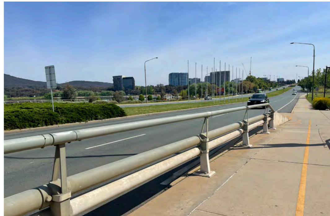
Figure 146: Current barrier termination.
