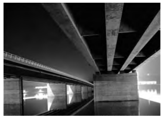
Figure 73: 1964. Kings Avenue Bridge 22.5.1964.
