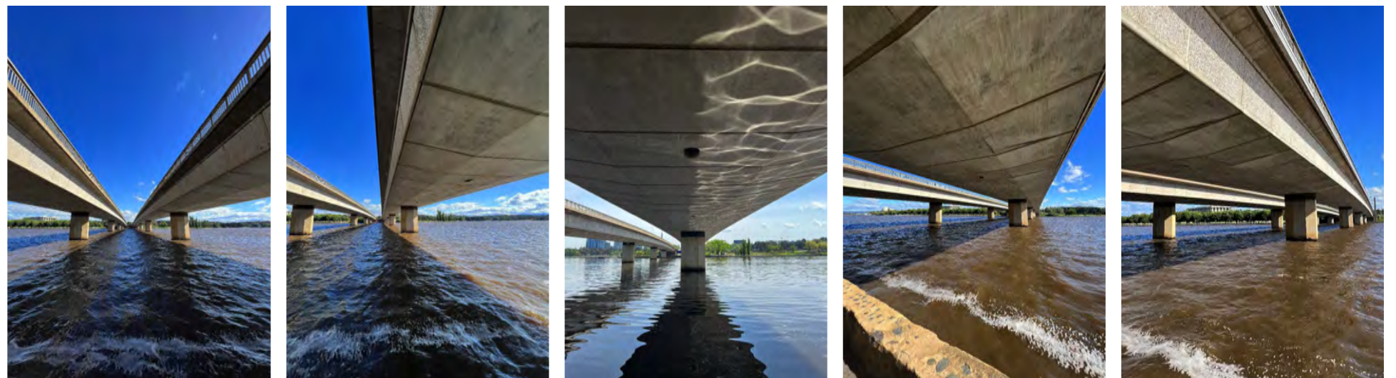
Figure 65: Different viewpoints under the northbound Bridge looking south
