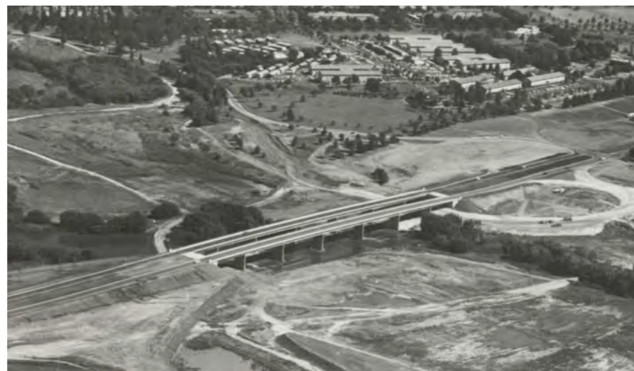
Figure 1: The Bridge was constructed in early 1960s
