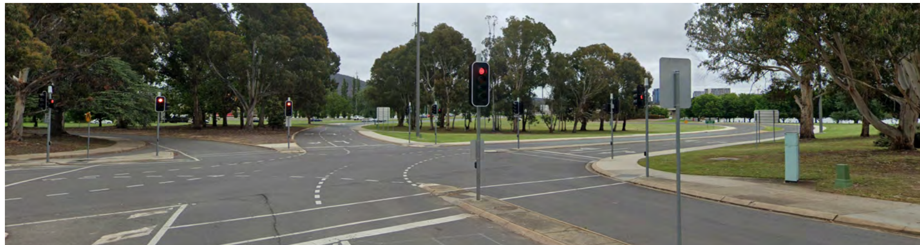
Figure 21: Intersection with Flynn Drive view from King Edward Terrace | Source: Google Earth
