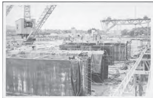
Figure 57: 1962. Commonwealth Avenue Bridge under construction, 1962 or 1963, 5 [picture]. Source: Trove, https://nla.gov.au:443/tarkine/nla.obj-145675273
