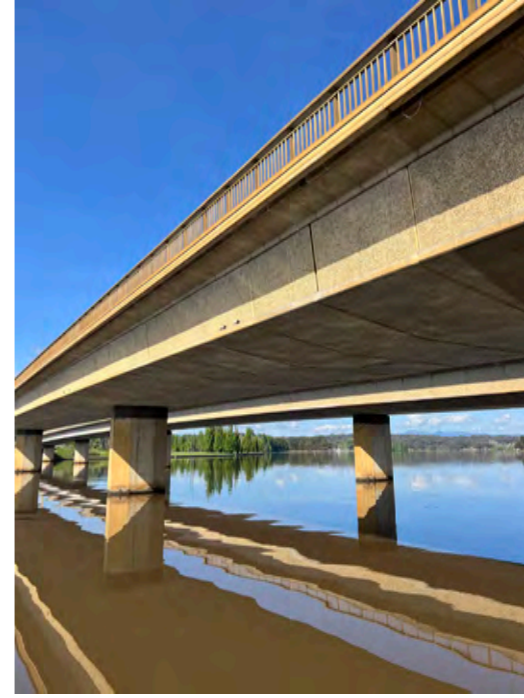
Figure 133: Detail shot of bridge edge showing precast panelling on eastern bridge.
