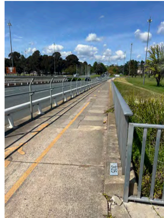
Figure 186: Flynn Drive bridge pathway.
