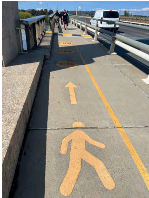
Figure 148: Pedestrian/ cycleway pinch point southbound.
