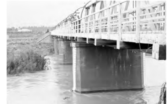
Figure 17: 1925. Commonwealth Bridge over the Monoglo River showing floodwaters and depth gauge. Source: National Archives of Australia, A3560, 3938, Item ID 3098112.
