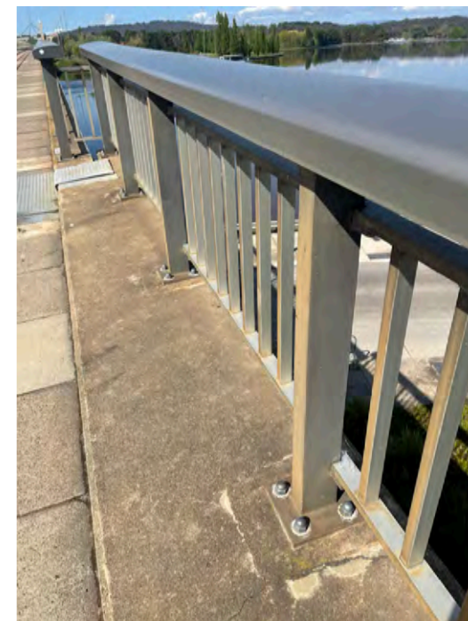
Figure 192: Balustrade detail.
