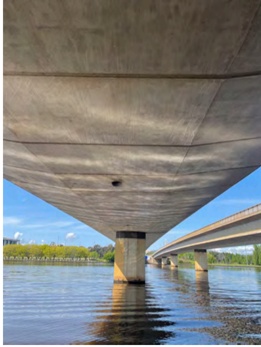
Figure 130: Centred view of eastern bridge soffit and pier.
