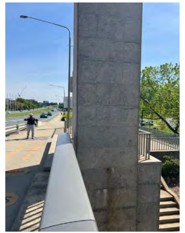
Streetlight adjacent to NE Pylon
