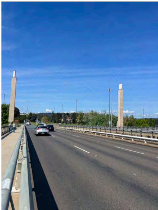
Figure 156: Southern Pylons viewed from southbound bridge.
