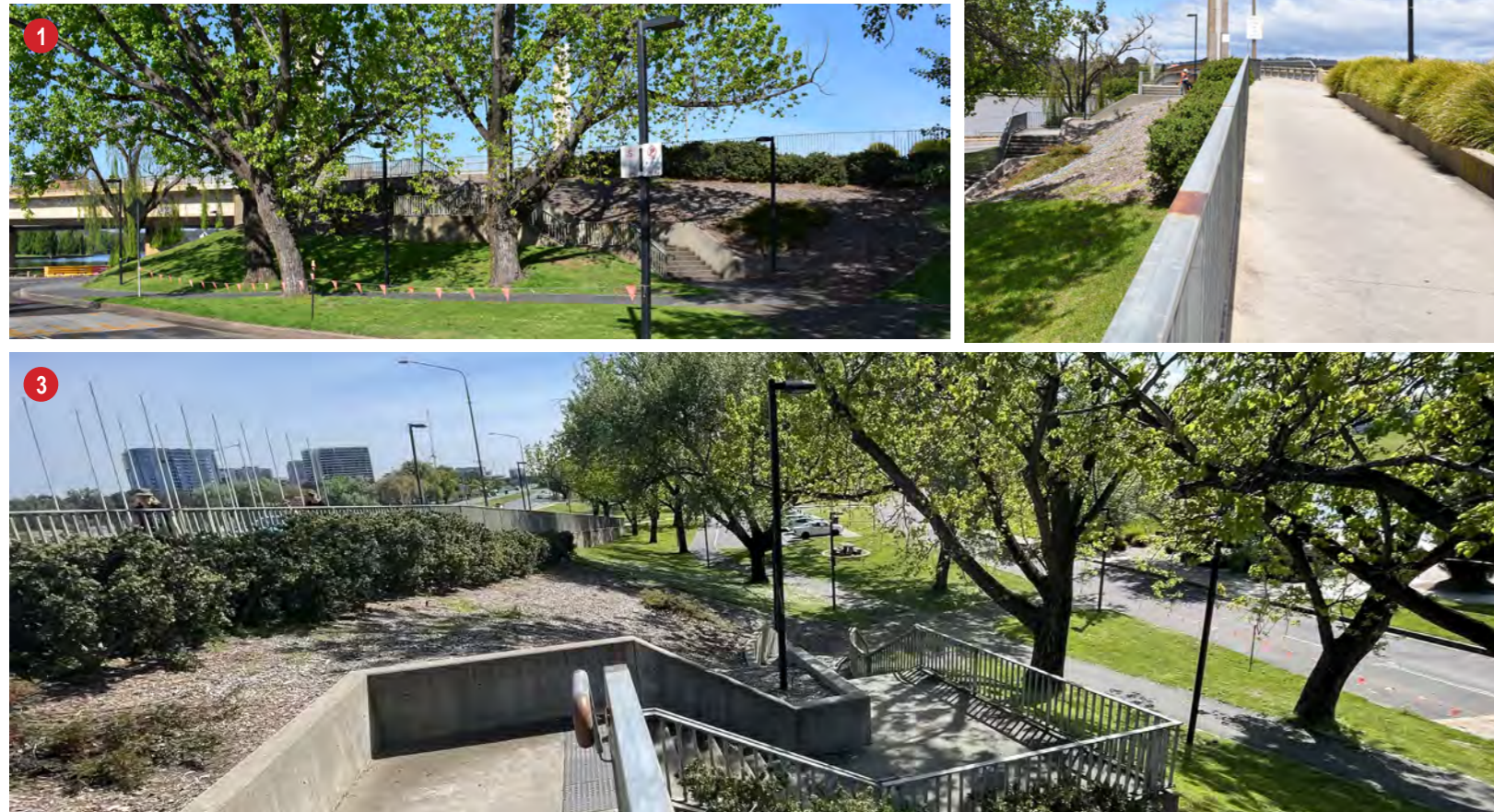
Figure 49: North-east approach existing site conditions
