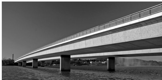
Existing view of external edge of bridge.
