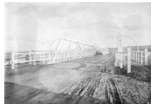
Figure 15: 1924. Completed Commonwealth Avenue Bridge looking south. Source: National Archives of Australia, A3560, 666, Item ID 3112248.
