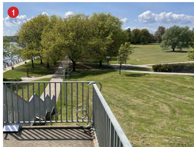
Figure 59: South-east approach existing conditions
