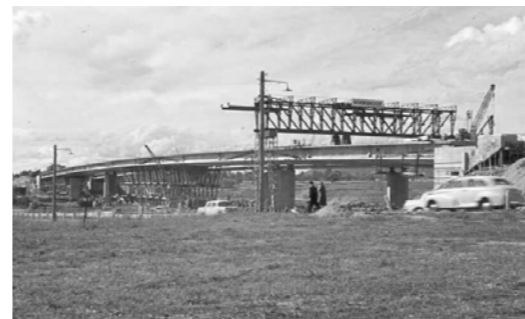
Figure 60: 1962. Bridge superstructure self supporting after post-tensioning. The timber falsework is in process of being removed. Source: National Library of Australia, nla.obj-143758408-1
