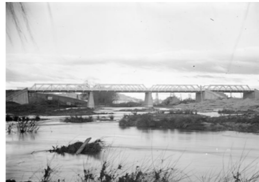
Figure 24: 1926. Commonwealth Avenue Bridge downstream from Molonglo River. Source: National Archives of Australia, A3560, 2079, Item ID 1964783.
