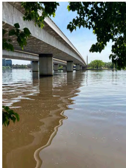
Figure 170: Bridge viewed from lake foreshore walk.
