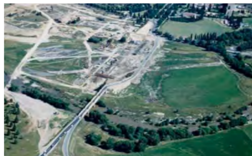
Figure 50: 1961. Commonwealth Bridge under construction December 1961.
