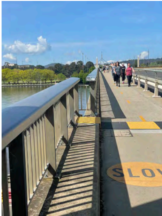
Figure 149: Balustrade junction on movement joint of bridge.
