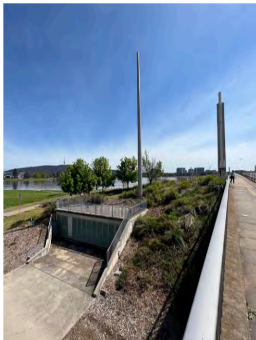
Figure 188: Substation on SW corner of bridge.
