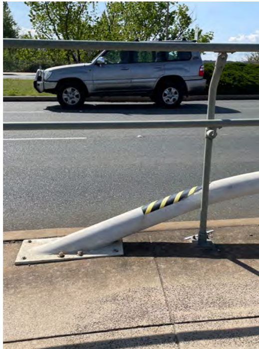
Figure 193: Termination detail of north bound barrier.
