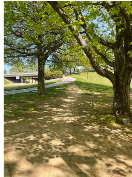
Figure 167: Desire lines coming off rammed path access to bridge.
