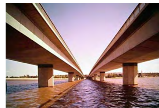
Figure 77: 1965. Commonwealth Bridge, Canberra. Source: National Archives of Australia, A1500, K12616, Item ID 11701647.
