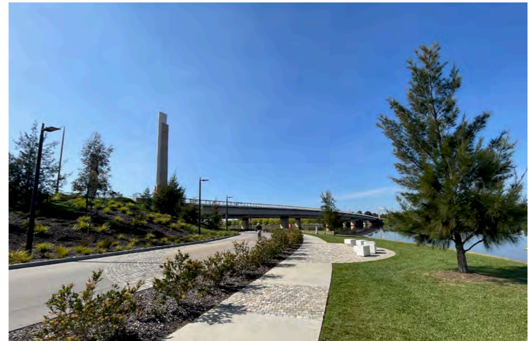
Figure 121: Commonwealth Avenue Bridge viewed from Barrine drive.
