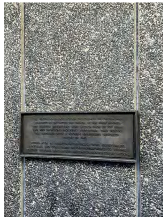
Figure 127: Plaque located between 2 bridges.
