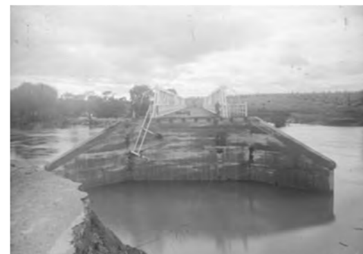
Figure 26: 1927. Commonwealth Bridge showing flood damage with the abutments washed away. Molonglo River in flood. Source: National Archives of Australia, A3560, 7668, Item ID 3238482.
