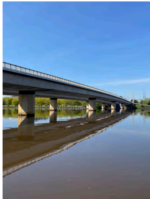
Figure 122: Commonwealth Avenue Bridge viewed from Barrine Drive looking towards Parliament.
