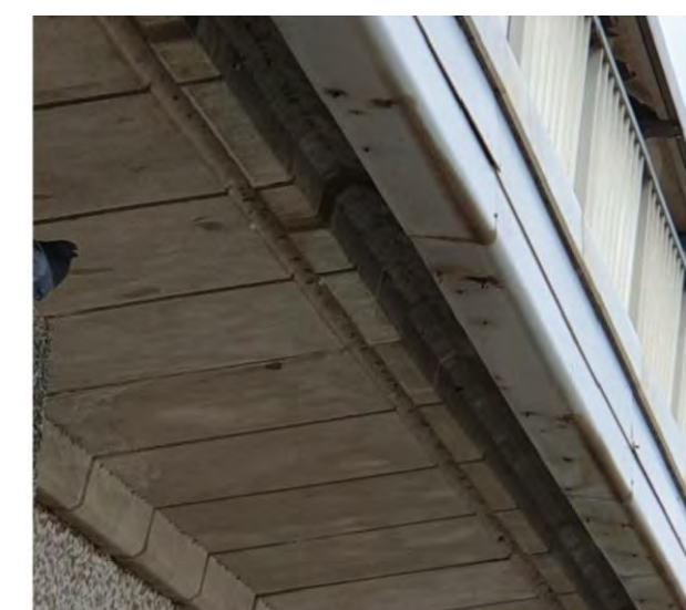
Figure 3.5 Commonwealth Avenue Bridge lighting in handrail and behind aluminium parapet cover to illuminate panels below. (Source: K Baker, 2020)
