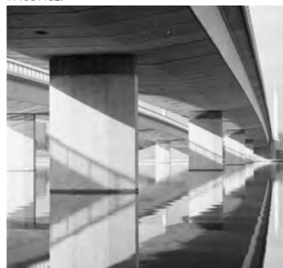
Figure 86: 1967. Commonwealth Bridge ACT - unusual angle looking between piles, Australian News and Information Bureau. Source: National Archives of Australia, A1200, L63643, Item ID 11202923.
