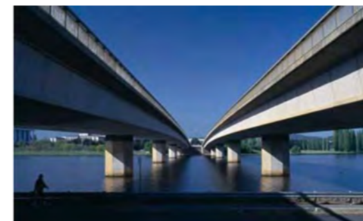
Figure 105: 1994. Canberra's Commonwealth Avenue Bridge. Source: National Archives of Australia, A6135, K6/1/94/163 Item ID 11721923.
