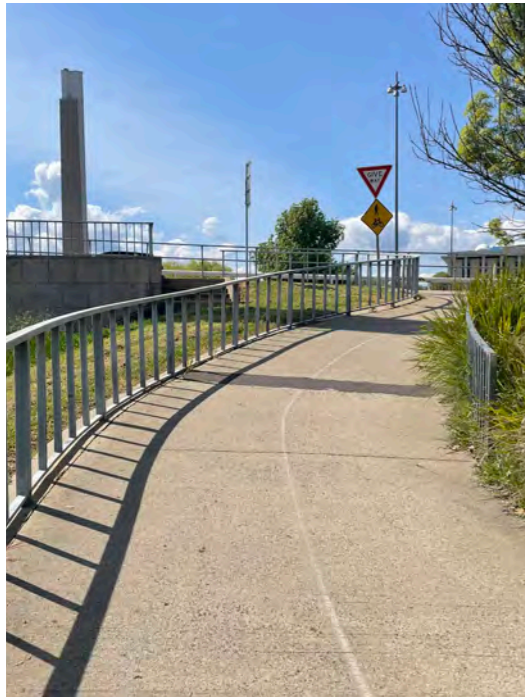
Figure 183: Connection from Flynn Drive cycle way onto bridge north bound.
