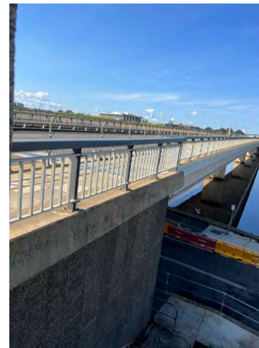
Figure 201: Edge detail abutment showing balustrade.
