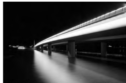
Figure 71: 1964. Commonwealth Avenue Bridge at night.
