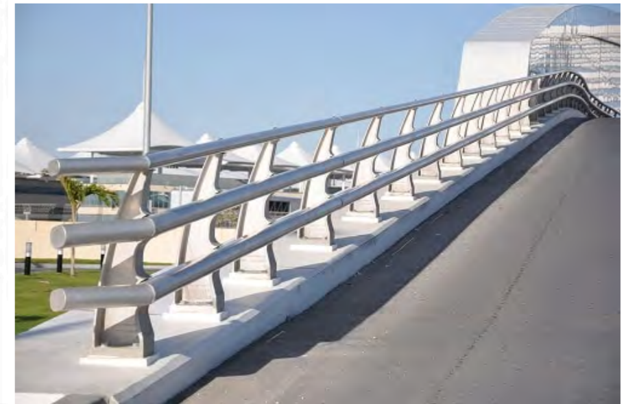
Minimum bridge barrier height varies with performance level.
