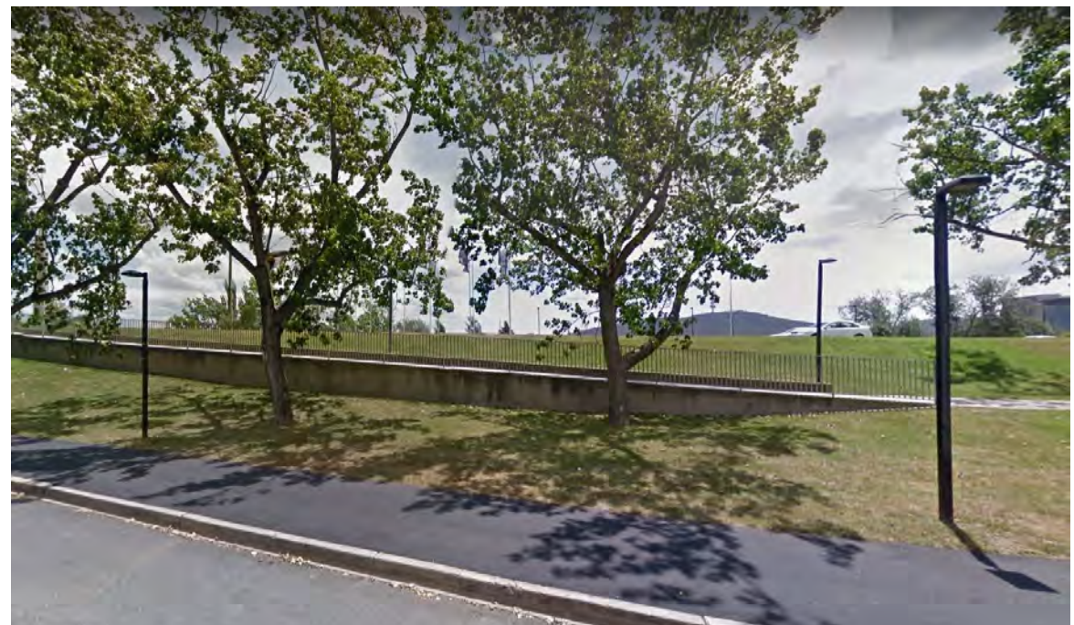
Existing Lighting on Barrine Drive
