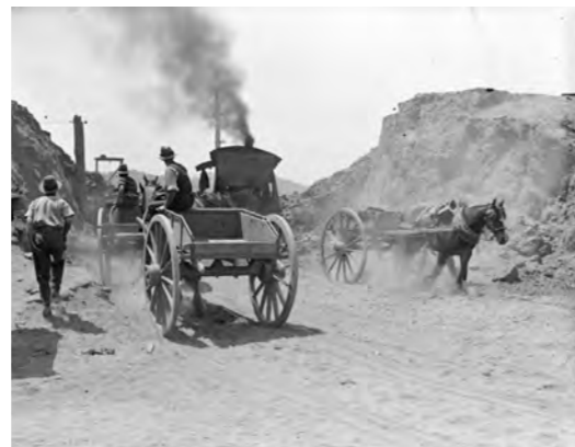
Figure 23: 1926. Keystone steam excavator at work on embankment of Commonwealth Avenue Bridge with horse drawn drays. Source: National Archives of Australia, A3560, 1326, Item ID 3119176.
