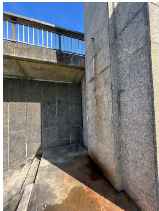
Figure 136: NE junction of bridge, stair and Pylon.
