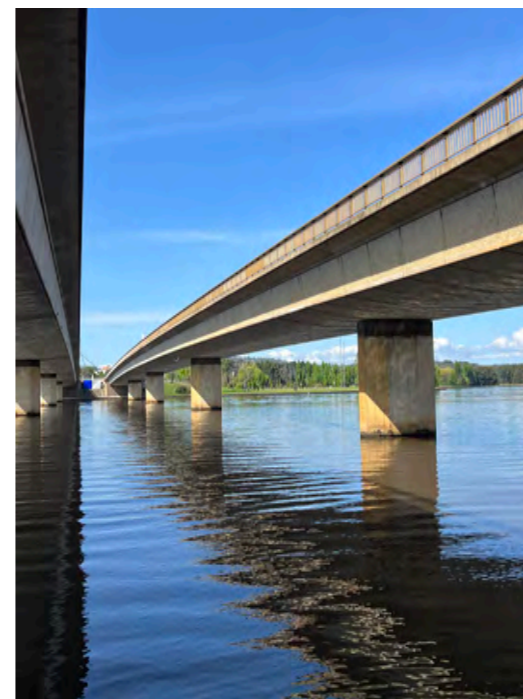
Figure 128: View of western bridge .
