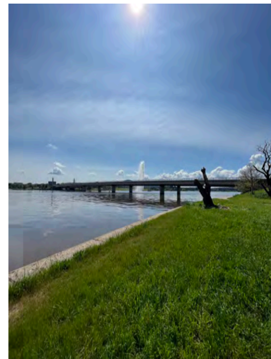
Figure 181: View of bridge from West Basin loop.
