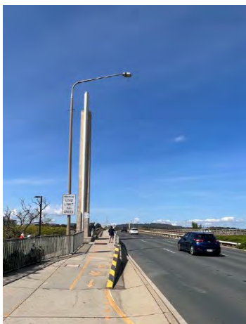
Approach to bridge Southbound
