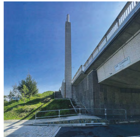
Current view of bridge abutment.
