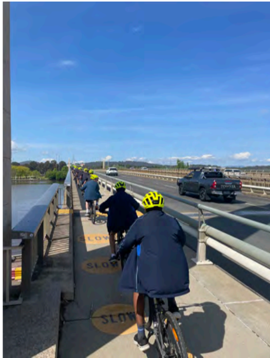
Figure 150: Pedestrian/ cycleway pinch point southbound.
