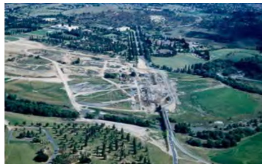
Figure 49: 1961. Commonwealth Bridge under construction December 1961.
