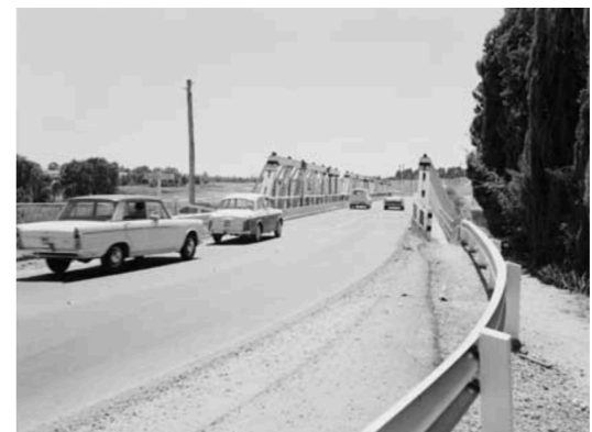
Figure 40: 1962. Site of accident on Commonwealth Bridge. Source: National Archives of Australia, A7973, INT630/1, Item ID 11715000.
