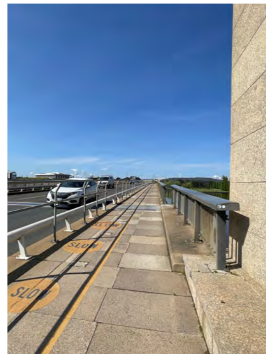
Figure 191: Pathway detail of pavement, barrier, balustrade and plinth.
