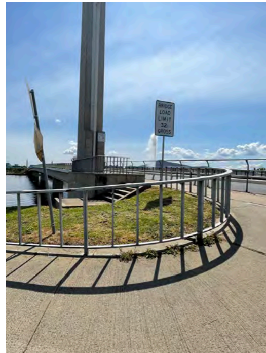
Figure 185: Connection from Flynn Drive cycle way onto bridge north bound.
