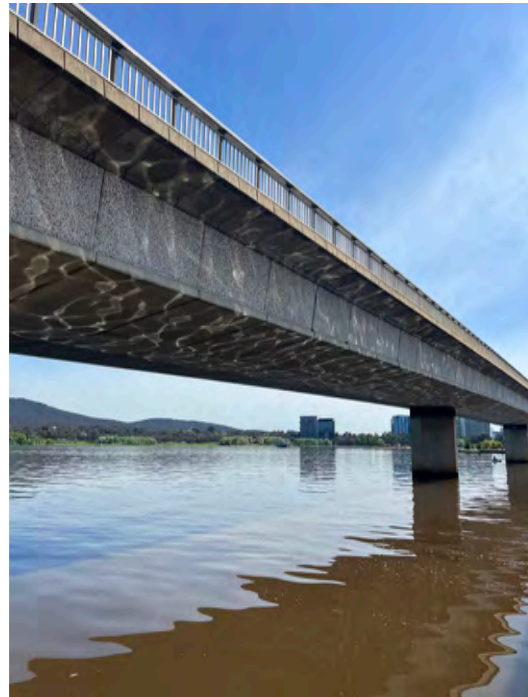
Figure 174: View of northbound bridge.
