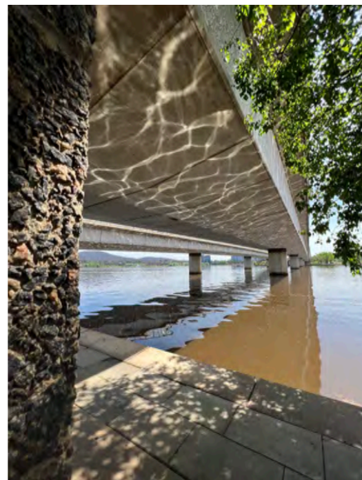
Figure 171: Detail bridge soffit with water reflection.
