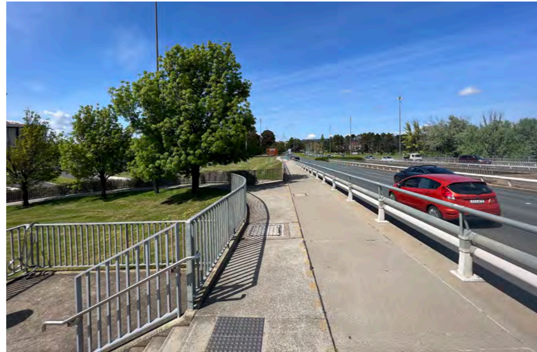
Figure 159: SE stair and ramp access to bridge.
