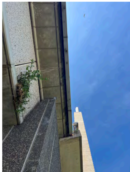
Figure 179: Detailed view of bridge connection and abutment.
