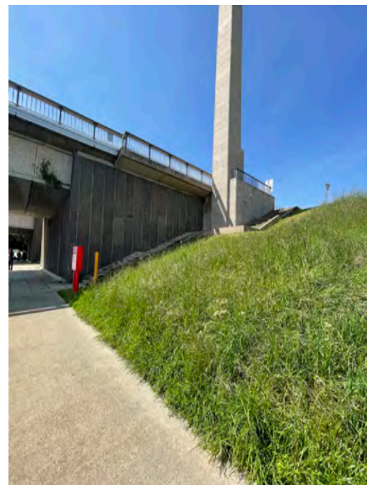
Figure 180: View of abutment.
