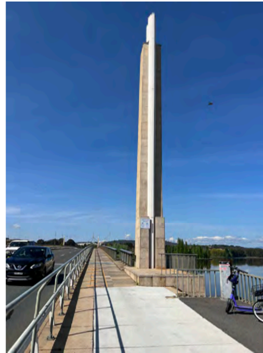
Figure 195: NW Pylon and pathway.
