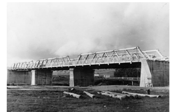
Figure 18: 1925. Commonwealth Bridge across Monoglo River, under construction Canberra, 1925. Source: National Archives of Australia, A1200, L83955, Item ID 11484929.
