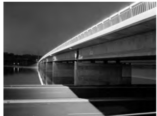
Figure 74: 1964. Kings Avenue Bridge 22.5.1964.
