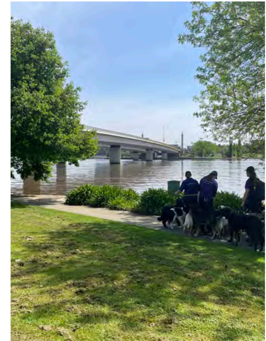
Figure 168: Commonwealth Avenue bridge viewed from oak tree avenue.
