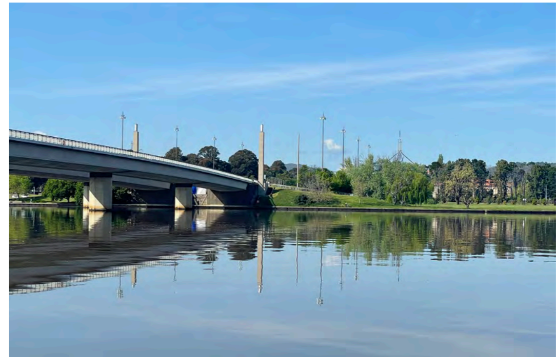
Figure 119: Commonwealth Avenue Bridge viewed from Henry Roland Park
