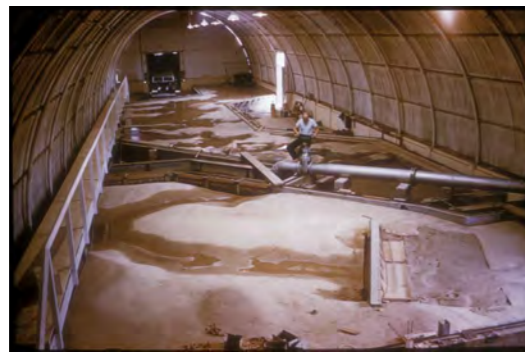
Figure 41: Hydrological scale modelling of the lake, with Scrivener Dam and bridges. Source: National Library of Australia, nla.obj-143692477.
