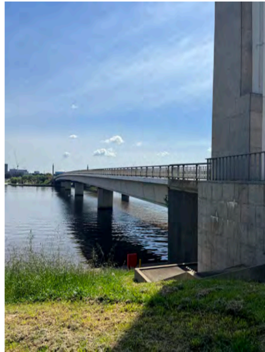
Figure 184: View northbound bridge.
