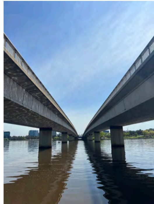
Figure 175: Looking north towards the City Centre.
