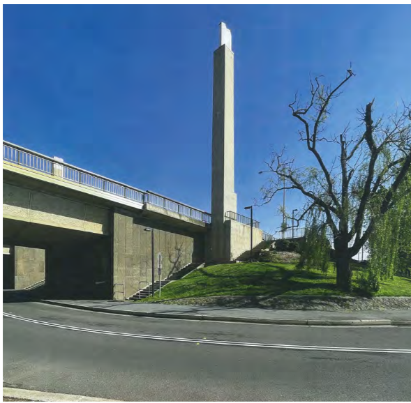
Current view of bridge abutment.
