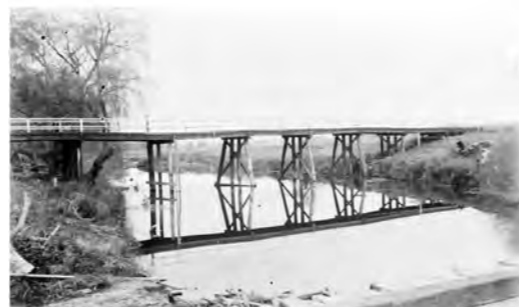
Figure 11: 1921-31. Temporary bridge while Commonwealth Avenue was being rebuilt. Source: National Archives of Australia, A3560, 662, Item ID 3112242.
