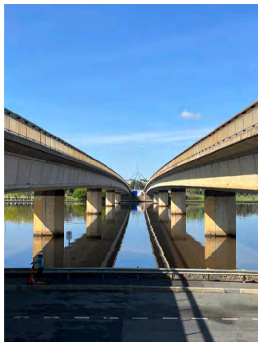
Figure 126: View from embankment between bridges towards Parliament House.
