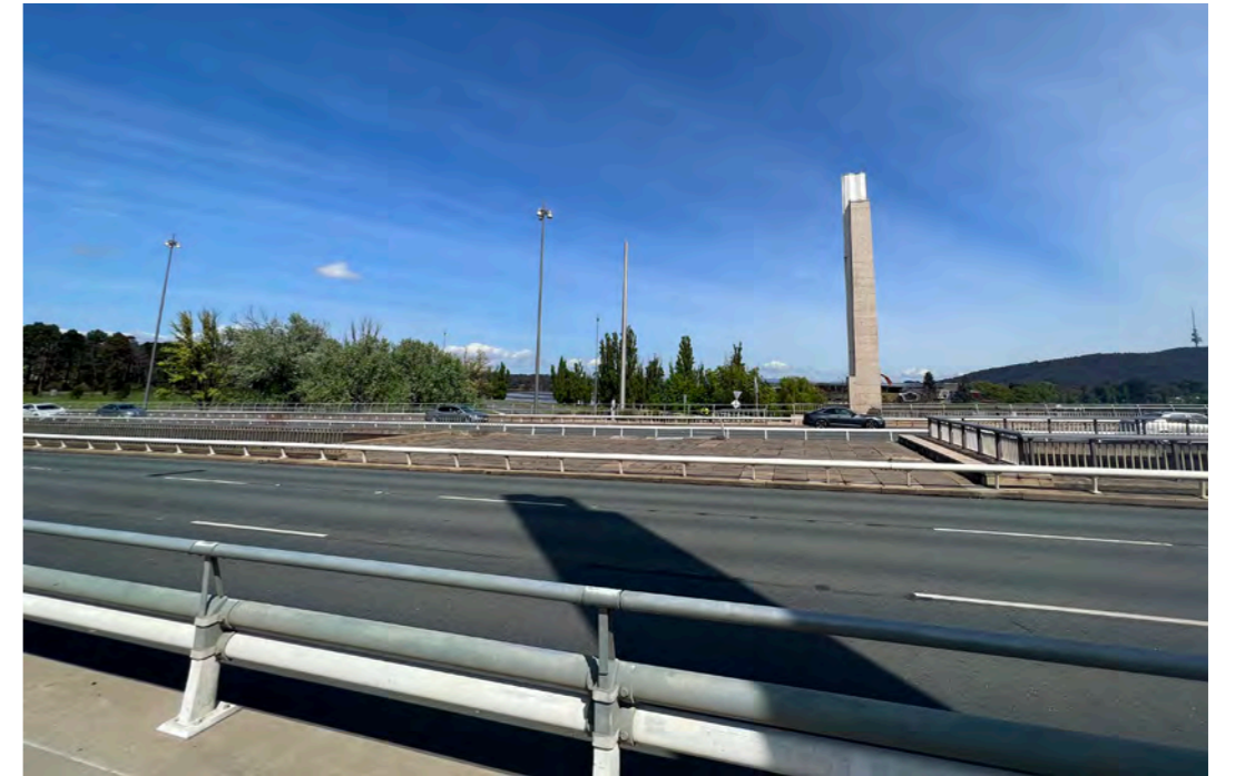
Figure 160: Section between Commonwealth Avenue Bridge and Flynn Drive bridges.
