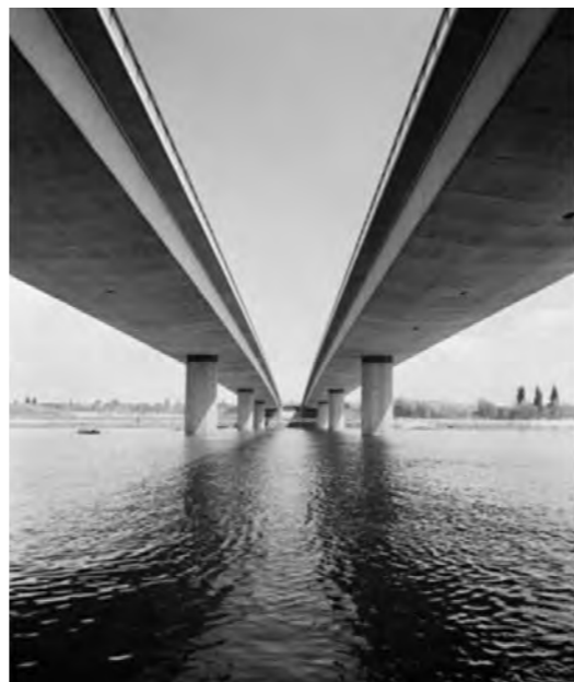
Figure 68: 1964. Commonwealth Avenue Bridge spanning Lake Burley Griffin, ACT.
