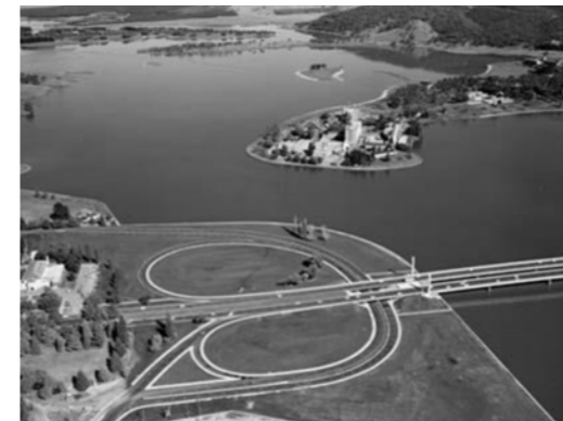
Figure 75: 1965. Aerial view of Commonwealth Avenue Bridge. Australian News and Information Bureau, photographer, W Nichol. Source: National Archives of Australia, A1200, L52723, Item ID 7594948.
