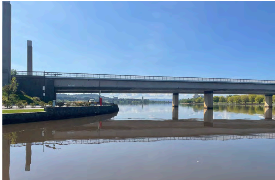
Figure 118: Commonwealth Avenue Bridge viewed from Henry Roland Park
