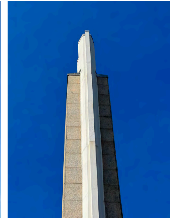
Figure 197: NW Pylon detail.
