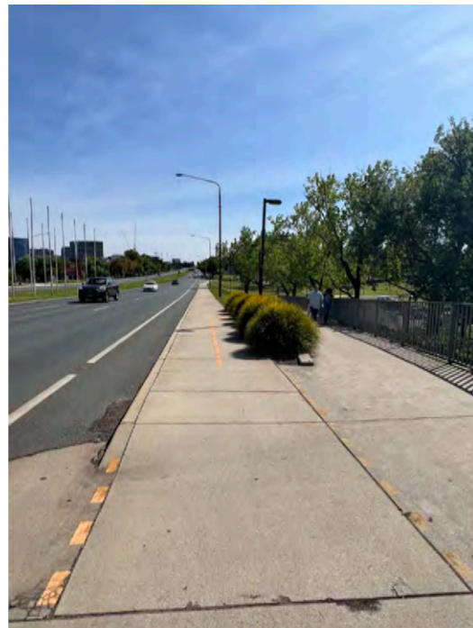
Figure 145: View of approach to bridge southbound.
