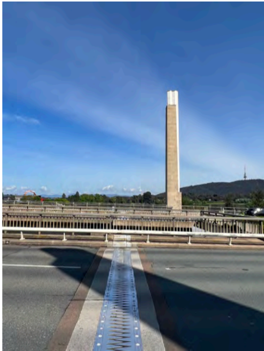
Figure 151: Movement joint of bridge looking west.
