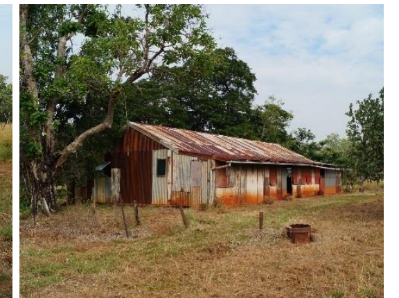
Old Goodparla - Structure
