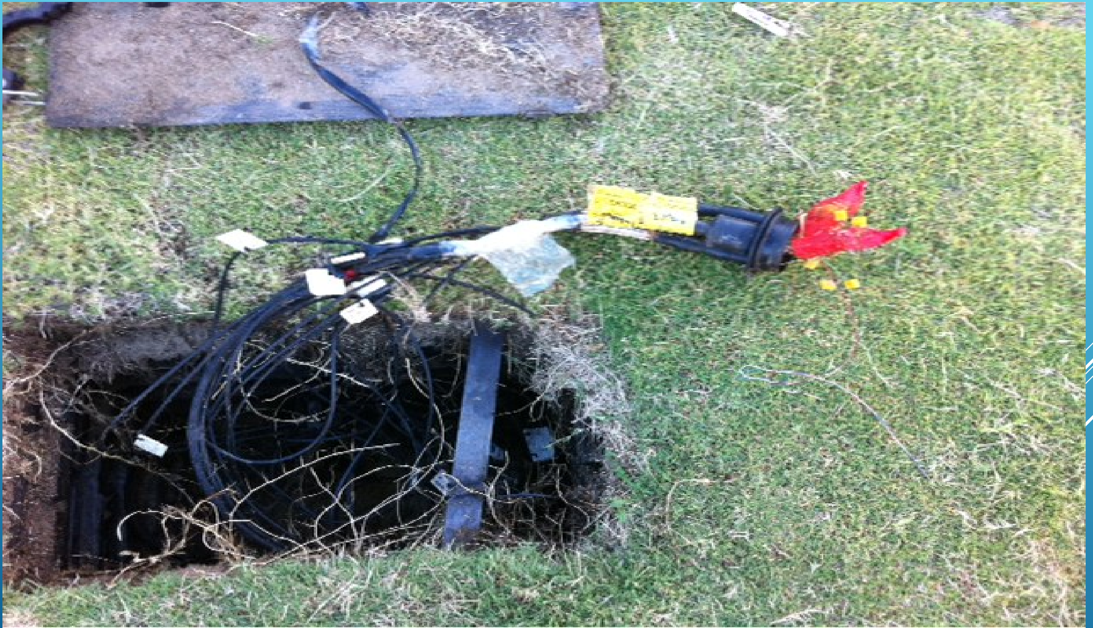
Photo: Energy in the network Project: Powerline GPS: 52.020000, 10.000000 Date: 2017-01-10 10:00:00
