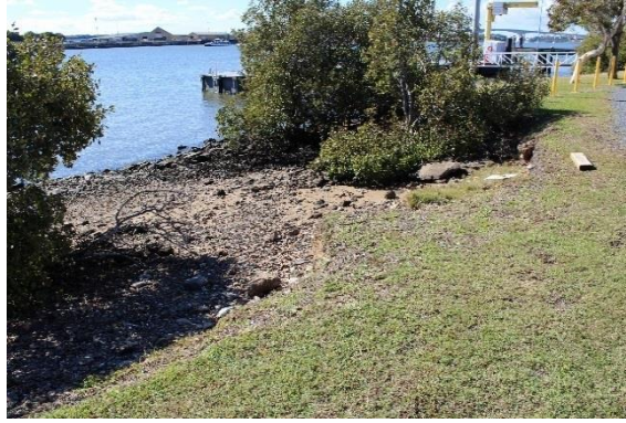
Figure 11: View of the current break, viewed from the landside. (GML 2017)
