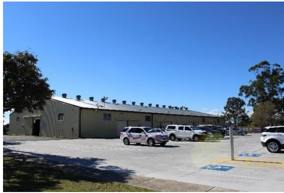
Figure 15: A002 and parking area viewed from the south-west. (GML 2017)
