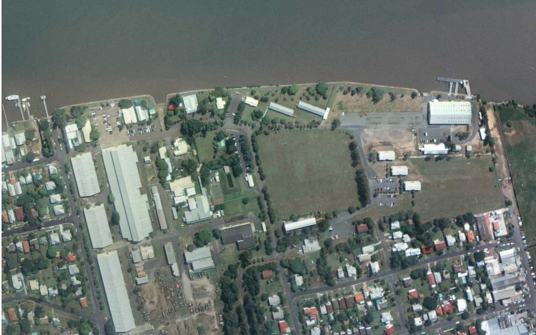
Figure B.44: 2000 aerial view of the site. The asset that was located on the western side of A002 has been removed by this time. (Source: QImagery Film QAP5738 Frame 142 Run 1, 20 April 2000)
