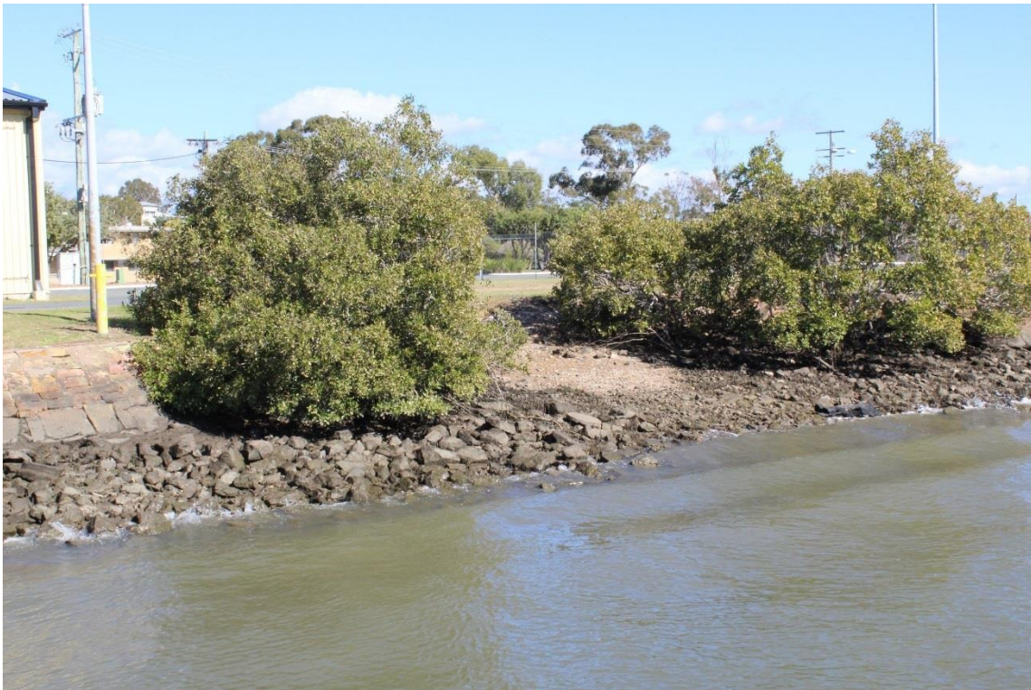
Figure 36: Current break in the sea wall where the proposed boat ramp will be constructed. (GML 2017)
