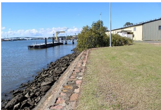
Figure 8: View along sea wall to A002 and the jetty. (GML 2017)
