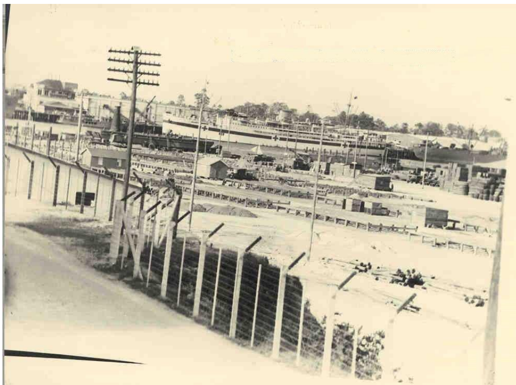
Figure B.16: Shed construction in progress in 1943. (Source: Oz@War website, Bulimba at war page)
