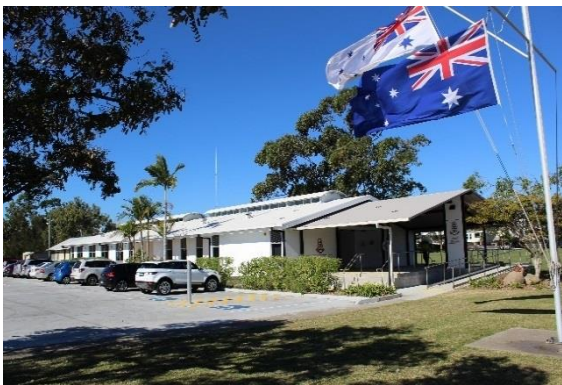
Figure 12: A008 viewed from the north-west. (GML 2017)
