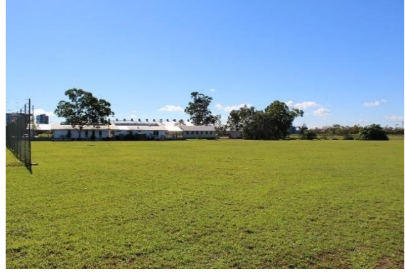
Figure 17: View across open area at the southern portion of HMAS Moreton, looking north-east. (GML 2017)
