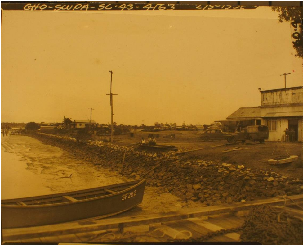
Figure B.13: US 1943 image along the Bulimba shore of the Brisbane River, prior to building removal works. The former J. Kitchen & Sons factory buildings are visible on the right side of the photograph. The rough stone sea wall can be clearly seen. (Source: Bulimba District Historical Society records)
