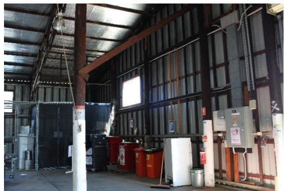
Figure 21: Timber support post detail, interior A002. (GML 2017)
