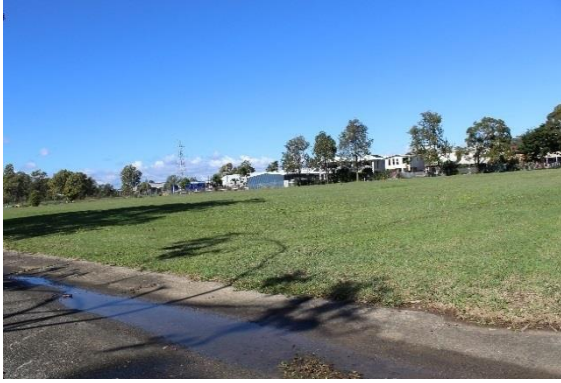
Figure 16: The current drainage swale on the southern side of A008 and A006, looking south-east. (GML 2017)
