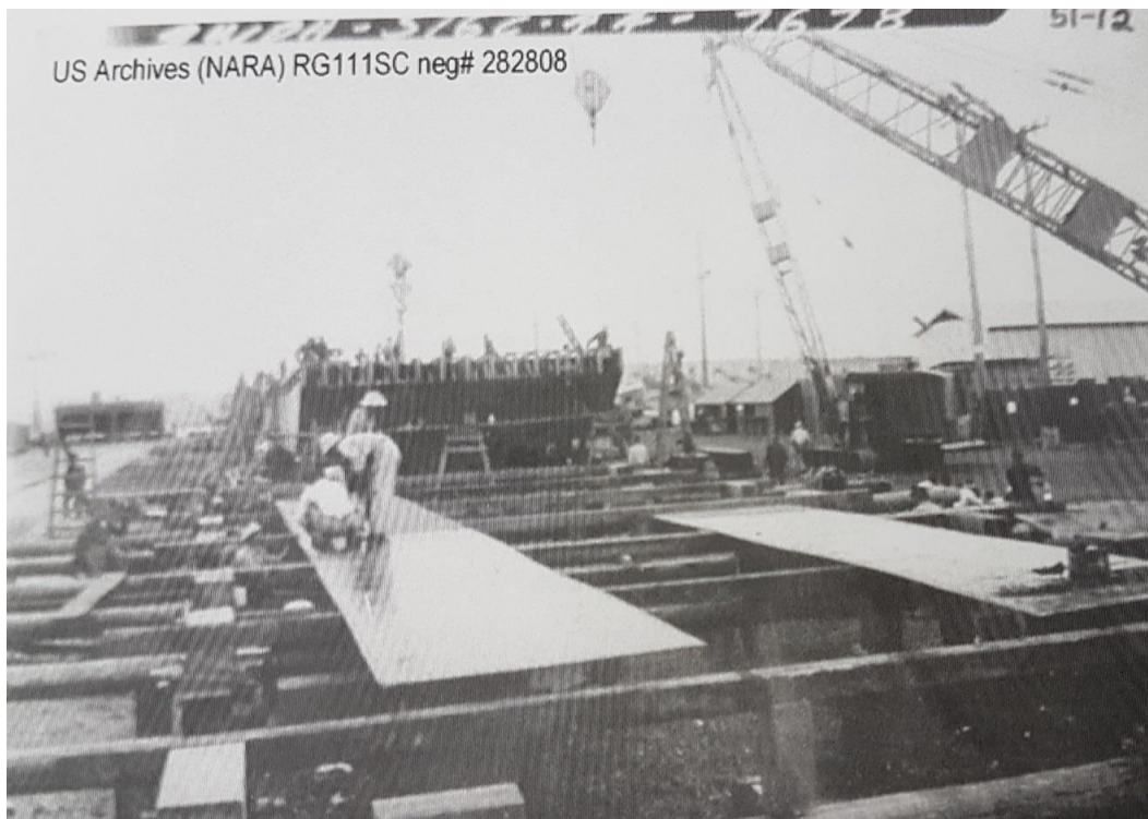
Figure B.20: Chinese workmen employed by the US Army lay the bottom plates of a kit form riveted barge at the Bulimba Ship Yards, Brisbane, 16 June 1944. The major parts of the barges, if not all materials, were factory cut to size and shipped from the US. These barges were crucial to the logistics of supply in the island campaigns of the Southwest Pacific. (Source: Marks & Dunn, undated, Brisbane WW2 v Now, No 7, copy held in the NLA)
