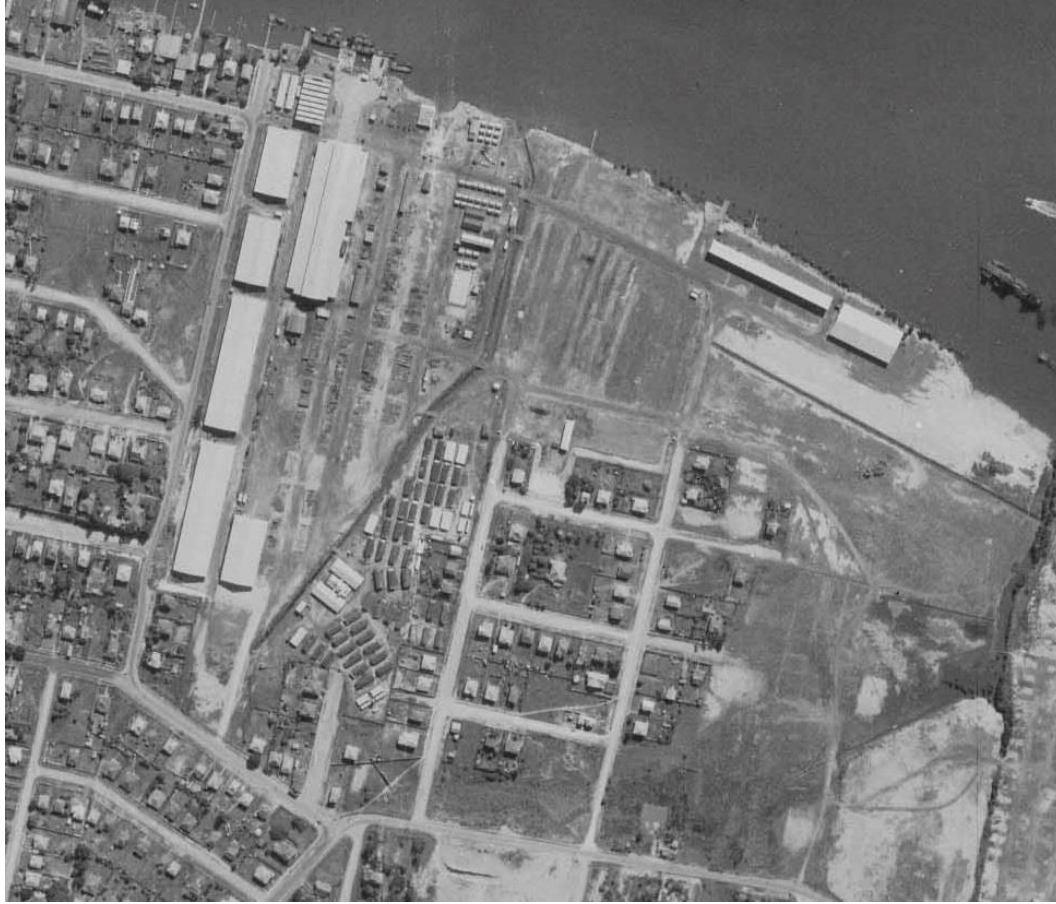
Figure B.29: Aerial view of the site in 1946. Asset A002 can be seen to the top right of this image. (Source: QImagery Film BCC2 Frame 34735 Run 9B 31 May 1946)
