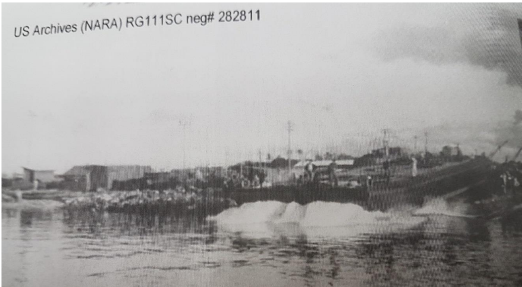
Figure B.22: Newly constructed barge, kit form riveted type, 102 feet 4 inches, slides off the ways at Bulimba Ship Yards, Brisbane, 16 June 1944. (Source: Marks & Dunn, undated, Brisbane WW2 v Now, No 7, copy held in the NLA)
