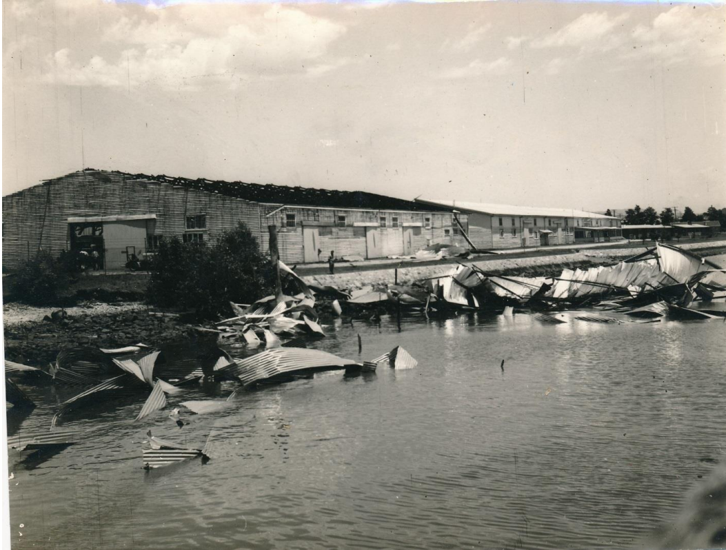
Figure B.37: Storm damage to A002 in 1973. Warehouse 5 adjacent to A002 can be seen in this image. (Source: Bulimba District Historical Society records)
