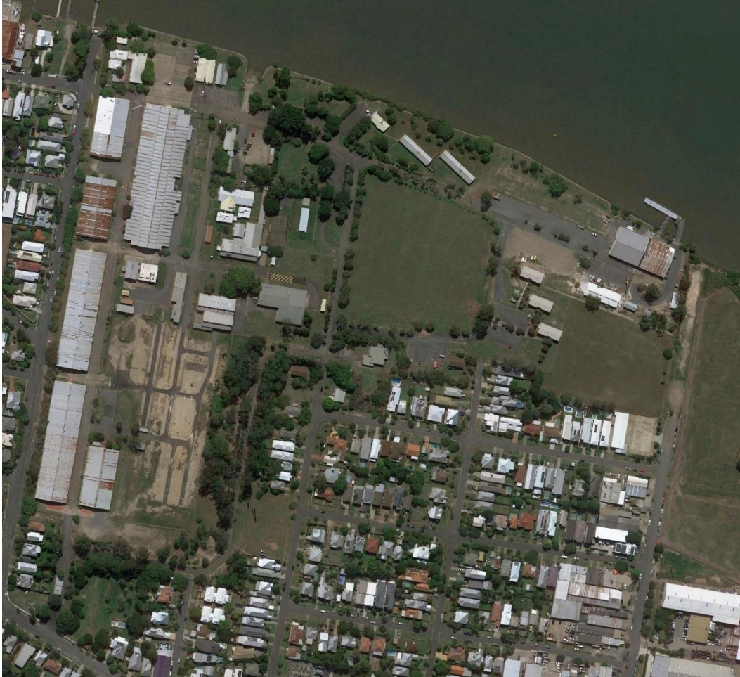
Figure B.47: 2015 aerial view of the site. The storm damage to the roof of A002 is evident in this image. (Source: Google Earth)
