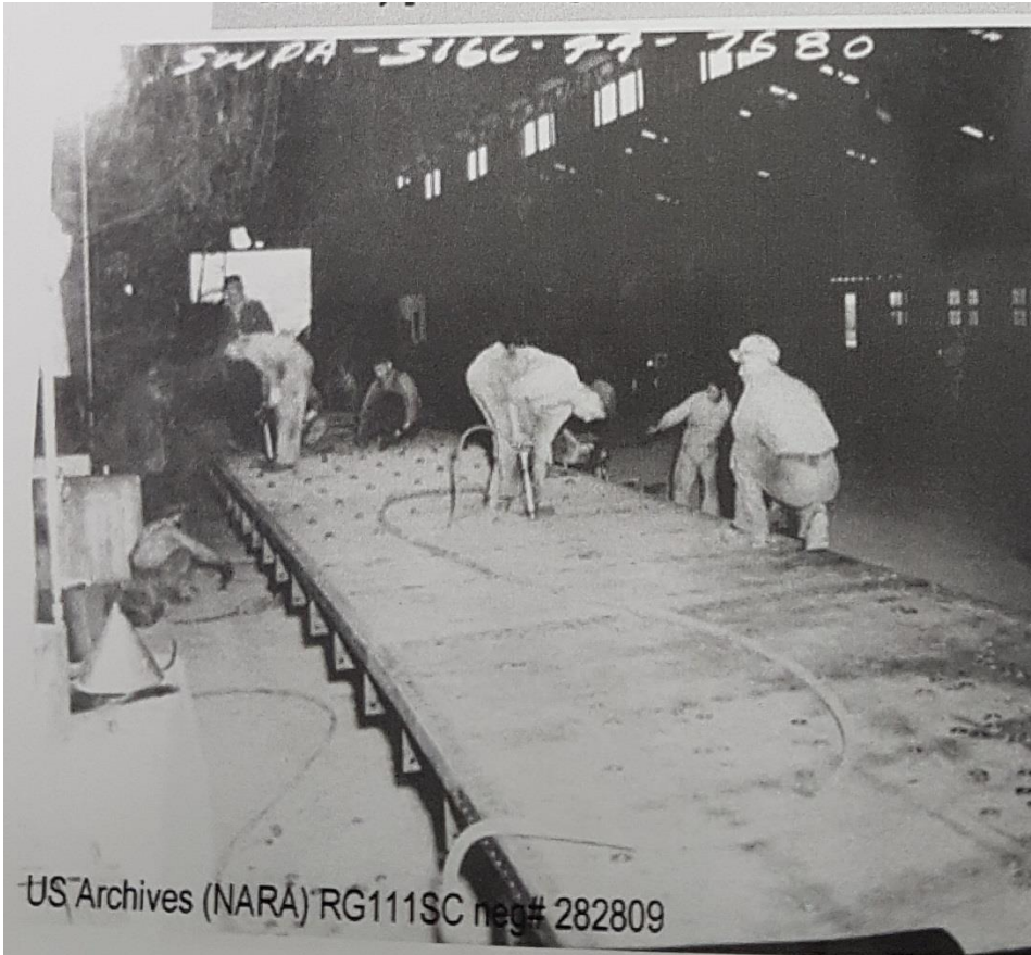
Figure B.21: Chinese workmen employed by the US Army prefabricate the sides for a kit form riveted barge 102 foot 4 inches at the Bulimba Ship Yards, Brisbane, 16 June 1944. Some work was indoors, but outside night lighting was used for shift work. (Source: Marks & Dunn, undated, Brisbane WW2 v Now, No 7, copy held in the NLA)
