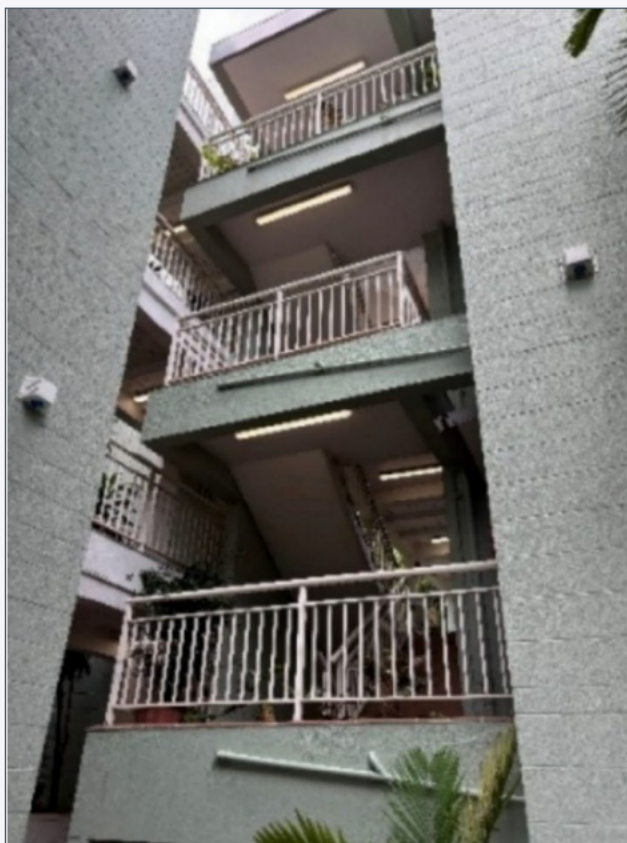
Apartments are connected by stairs across 7 levels.
