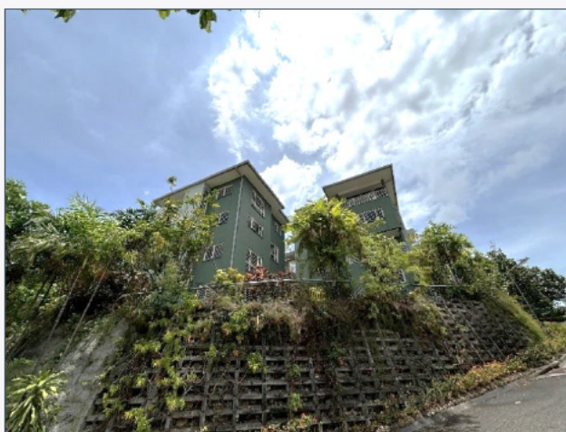
Retaining wall showing typical topography.
