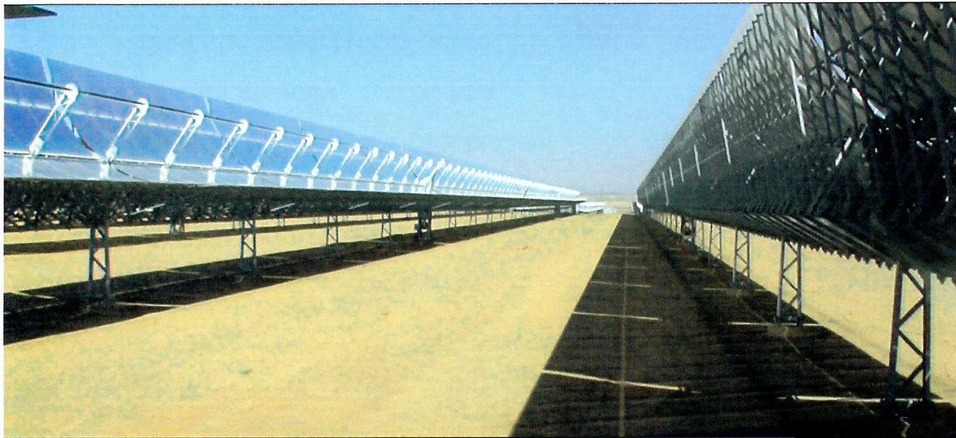
Andasol 3 a Typical Spanish 50MW<sub>e</sub> trough plant
