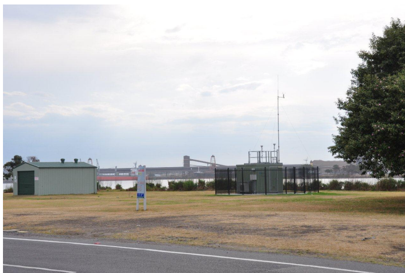
Orica Air Quality Monitoring Station Stockton
