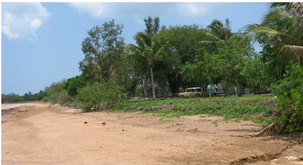
Fig F.4 Looking north showing how the road at low area #1 is only 1.2 m above the HAT level of 4.0 m AHD.
