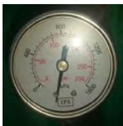
This is a photo taken of gauge at isolation 25.11.15
