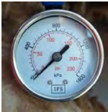
This is a photo taken of gauge at isolation 25.11.15
