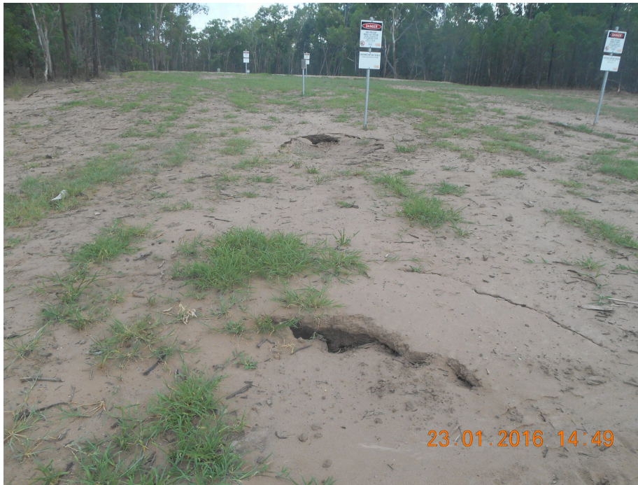
Subsidence along the gas pipeline photo courtesy of local resident
