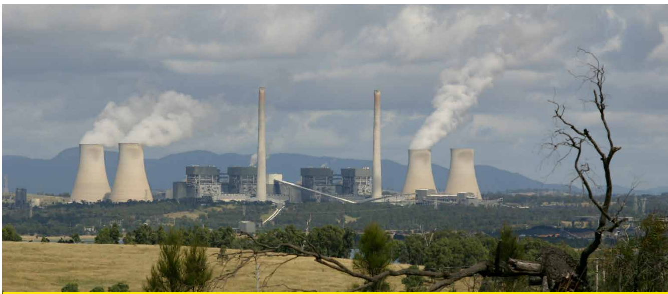
Hunter Valley coal-fired power station. Credit Donna Green
