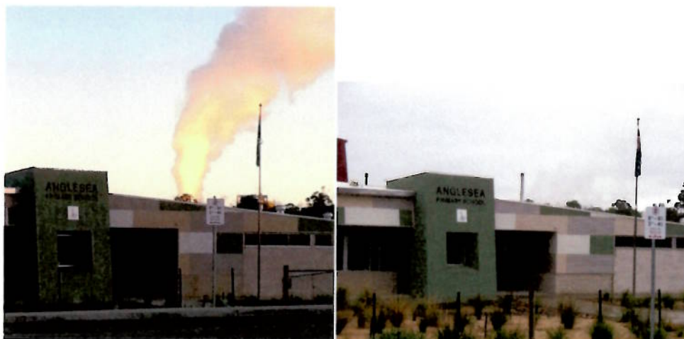
Photos 1 (left) showing cooling tower steam plume and 2 (right) actual power station stack
