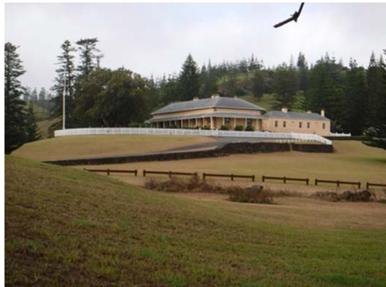
The Administrator's palace...next to the golf course.
