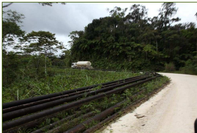
Pipelines of an existing oil facility around Lake Kutubu Credit: Damian Baker
