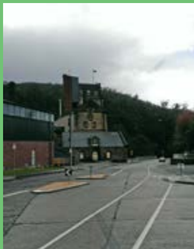
Hobart City Council has installed a pedestrian refuge on Strickland Ave at Cascade Brewery and included an uphill bike lane as part of the project. This short link provides a connection for bicycle riders using the Hobart Rivulet path from the Cascade Gardens to the Old Farm Road turnoff.
