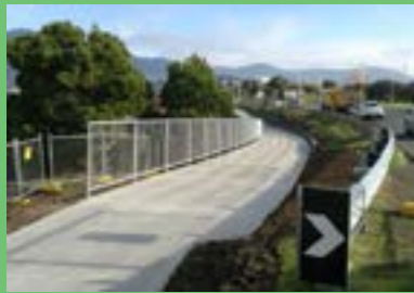
Before and after photographs of the Eastern approach to the Tasman Bridge. This 400m shared pathway was co-funded by Clarence City Council and the Department of State Growth. It improves cyclist and pedestrian access and creates a safe, off-road link to an overpass that leads to a local high school.
