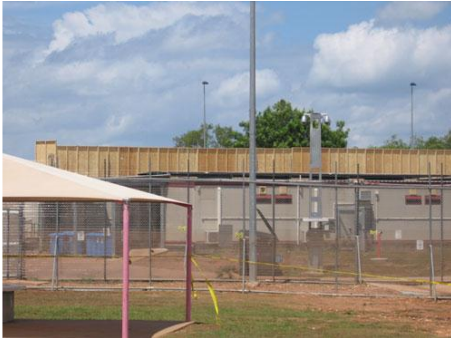
Electrified fence separating North and South compounds, Northern IDC, September 2010.
