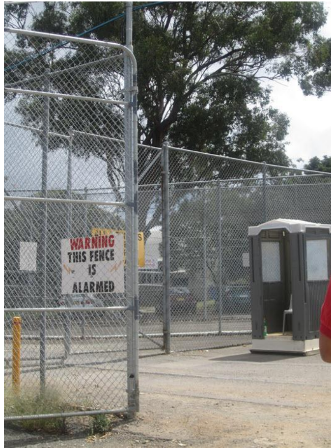
External fences, Villawood IDC, February 2011.
