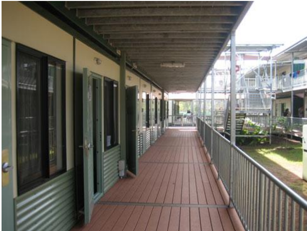
Offices and accommodation, Darwin Airport Lodge, September 2010.
