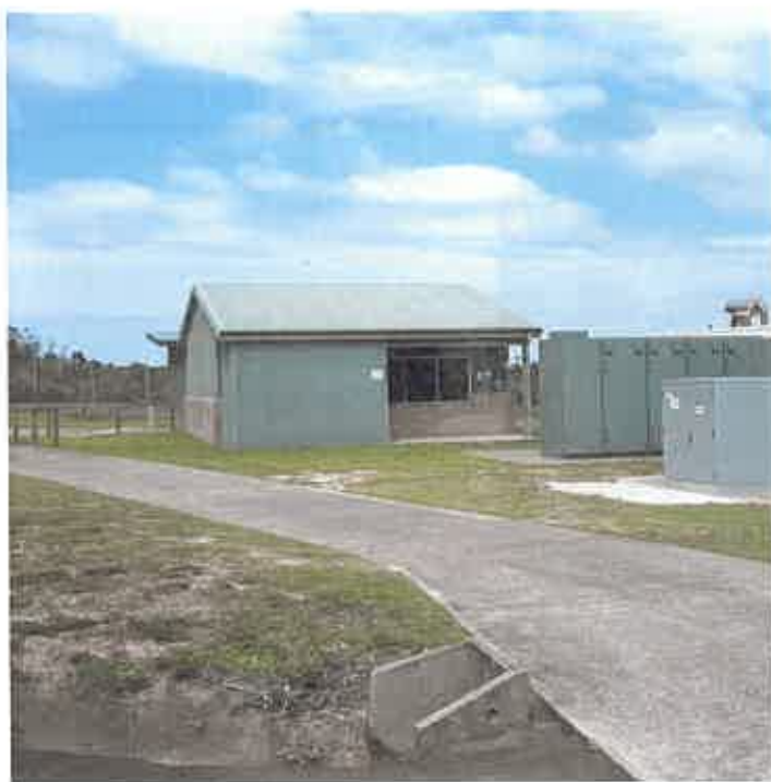
Figure 1 – Existing MTF at RANSSSS East, HMAS Creswell
