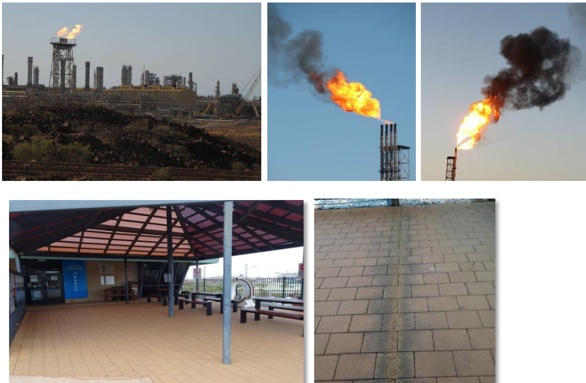
Figure 5. Emissions from the Woodside industrial plant on Burrup Peninsula (above), photograph of Woodside Visitors Centre showing small gap between two roof lines (lower left) and degradation of paving bricks where rain falls between the two roofs, with the dark colour suspected to be from microbial growth adjacent to the erosion line (lower right).
