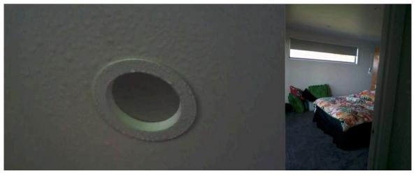
Figure 19: An example of what happens when there is thermal bridge between mid-roof temperature and living dew point: condensation around the uninsulated downlight.
