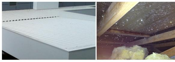
Figure 24: The constantly wet, and often dripping underside of the roof.
