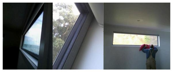
Figure 17: An example of what happens when there is thermal bridge between site temperature and living dew point: condensation on the aluminium frame of a south facing window.
