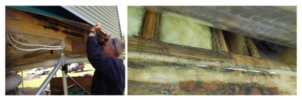
Figure 16: Often the true effect of condensation happens inside the wall framing. A builder helps dismantle the sheet metal cladding that is hard fixed against the studs (no battens) causing the wrap to be thermally bridged with the cold exterior. Indoor vapour, unable to pass through the foil wrap condenses on the insulation which acts as a reservoir, keeping the studs and bottom plate a moist breeding ground for mould.
