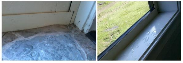
Figure 29: Condensation forming on the kitchen flooring due to poorly installed insulation and a vapour impermeable vinyl finish. Around the window reveals the thermal bridging of the structure results in condensation.
