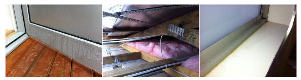
Figure 2: New house in Launceston 5 months after occupation. Photographs supplied from builder who would like to remain unnamed. Copious condensation forms on door and windows. However it is only upon prying open the roof is the extend of mould growth appreciable.
