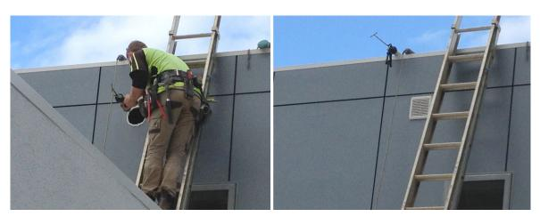
Figure 23: Installation of roof ventilation, In total 4 of these vents were installed.
