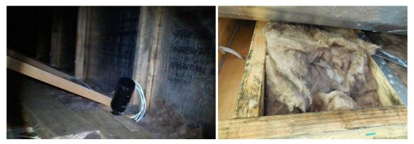
Figure 31: Inside the roof and walls where there is extensive condensation and mould growth on the timber strucure in the house that has been occupied for about 2 months.
