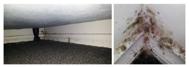
Figure 30: Under the bed, the wall and carpet have limited exposure to the heating and experience thermal bridging to the external walls.
