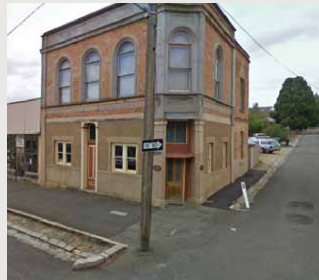
Lane connecting units to main street
