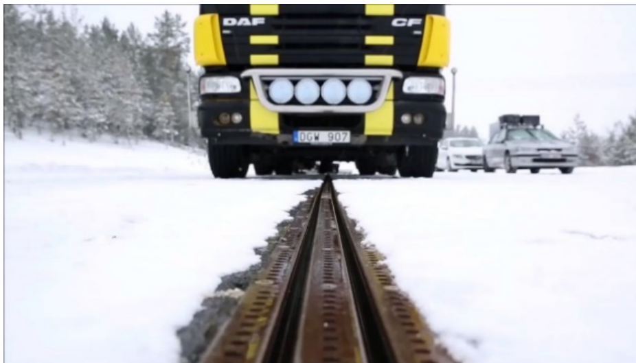
Figure 56: Charging Rail In Road (Source: independent.co.uk )
