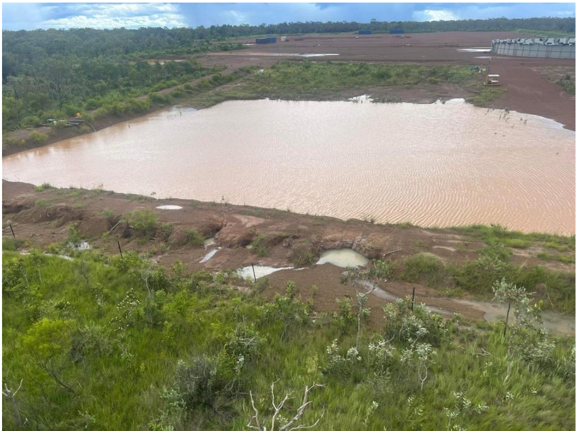
Courtesy Protect Big Rivers 4 Bund wall giving way on Maverick well pad, known site of contamination.
