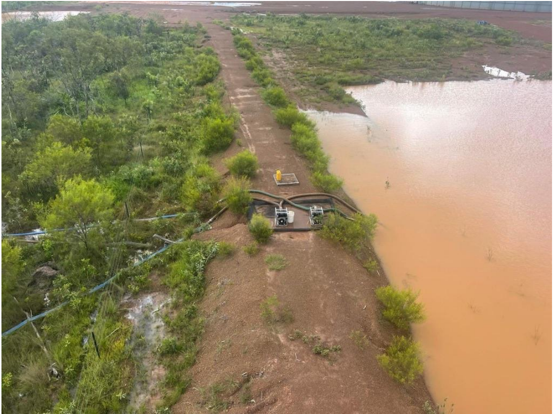
Courtesy Protect Big Rivers 5 Pumping over the bund wall from Maverick, known site of contamination, Tamboran.
