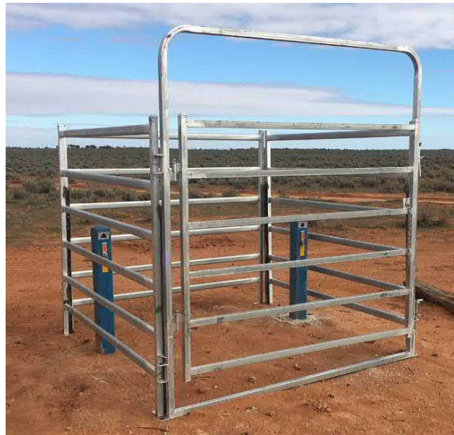
Figure 31 Bore headworks completion at W02S and W02C
