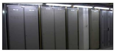
This (above) is a typical installation of several racks<sup>16</sup> of (iiNet) DSLAM equipment all in physical competition with Telstra, Optus and other DSLAM equipment, all in the one in a (Telstra) metropolitan exchange site, and separate Points of Interconnect.
