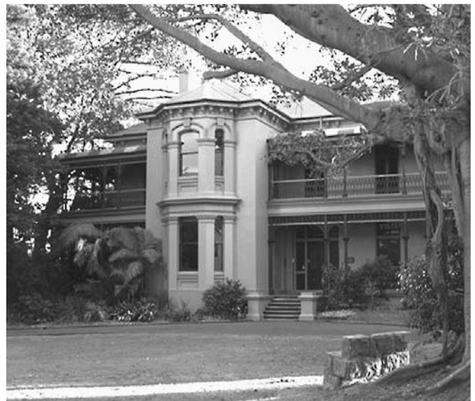
Scarba House as it is today
