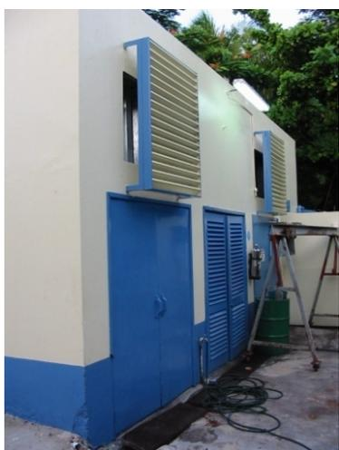
*It is recommended that a purpose designed generator shed be used, however if the proposed existing shed is used, add acoustic louvres and use a residential level exhaust muffler to enable maintenance of the natural soundscape around Mutee heads. These louvres are quite cheap.*
