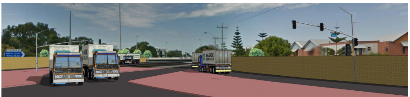
Figure 18. A before and after shot of the intersection of Tydeman and Stirling in North Fremantle. High sounds walls and wide turning radii allow 80 km per hour truck movements with light priority through this narrow urban area.
