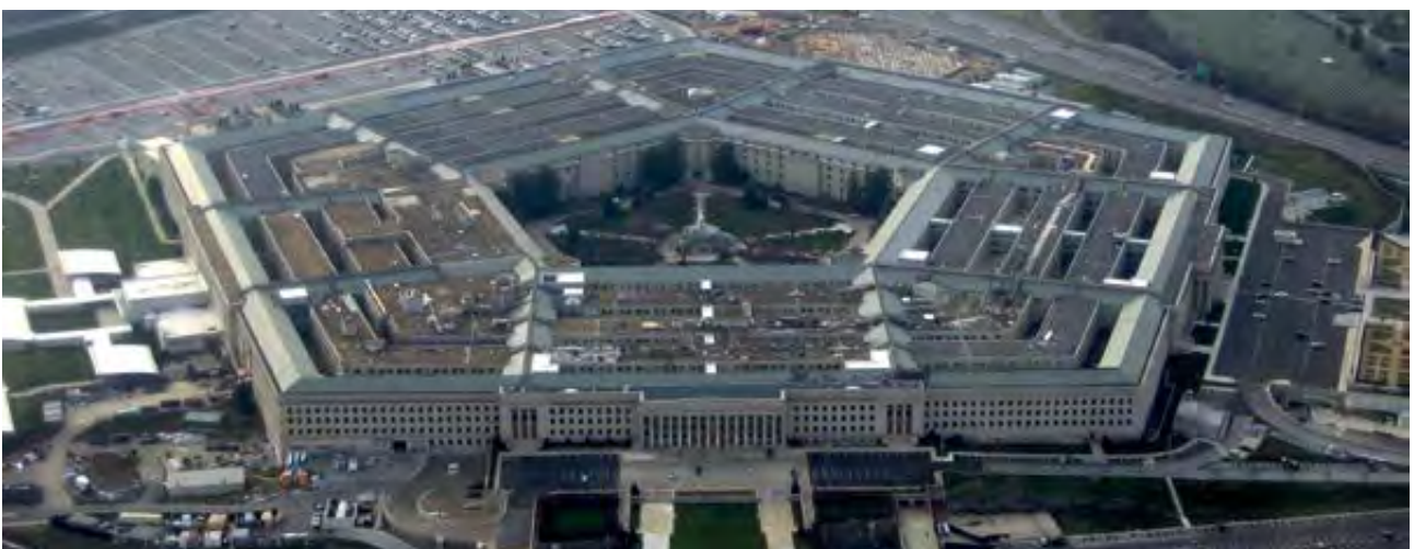
Figure 28: The Pentagon as seen from the air. The US Department of Defence considers climate change to be a significant threat to national security.
