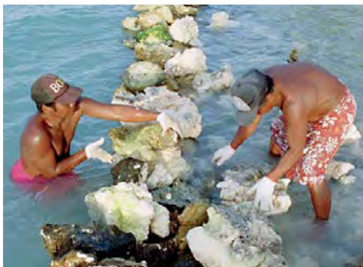
Figure 23: Residents of the low-lying Pacific island of Kiribati use coral rocks to build temporary walls in an attempt to break the swell of increasingly large king tides.
