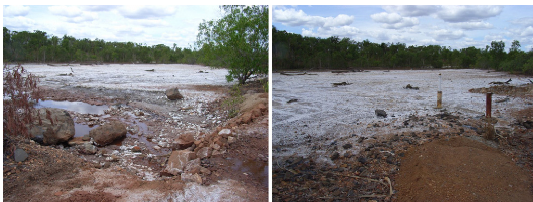
Fig. 7. Former Sweetwater Dam, July 2007; Note – the water and flow in the left photo is continuing seepage from White's waste rock dump (see Fig. 3) (photo's G M Mudd).
