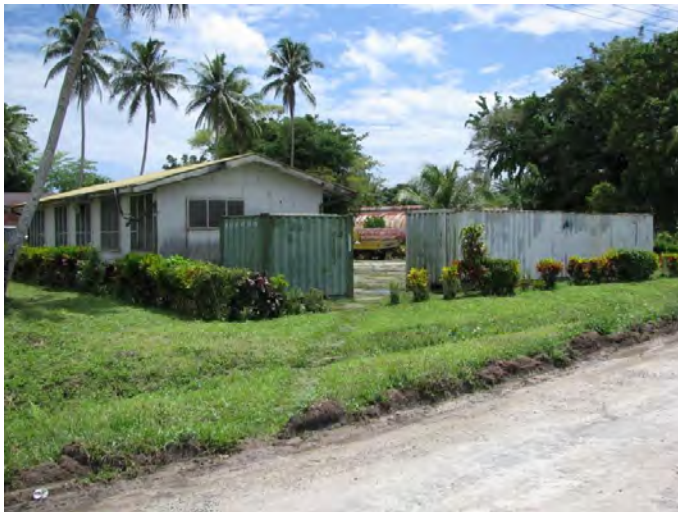
Figure 3 Greenfield South (SKM, 2013)
