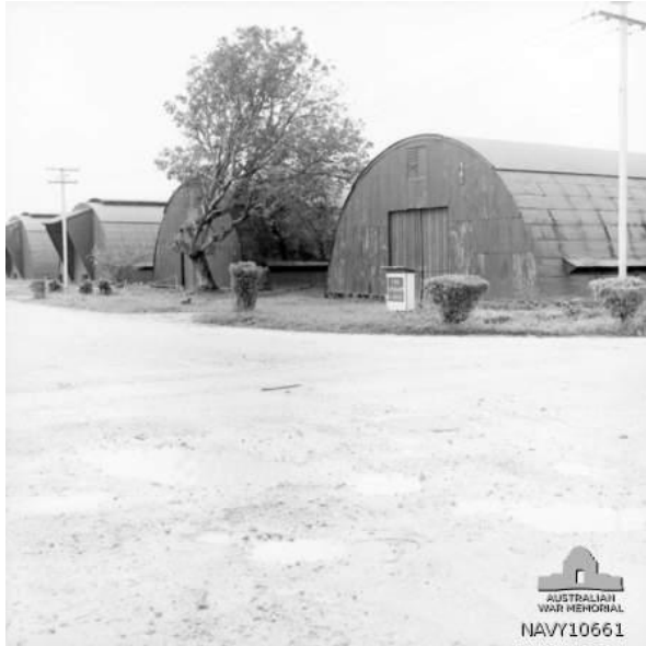
Figure 18: Nissen (or Quonset) Huts at Lombrum Point c 1950 (Source: Australian War Memorial)
